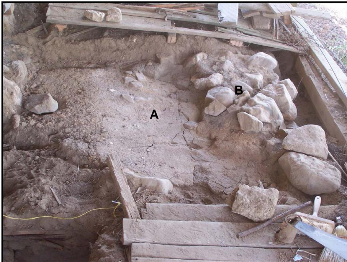
**Figure 88: An area of the original porch cleared of debris. Note the hard packed earthen surface that appears to have been laid as a mud slurry (A) and the shallow cobble footing along the north edge (B).**
