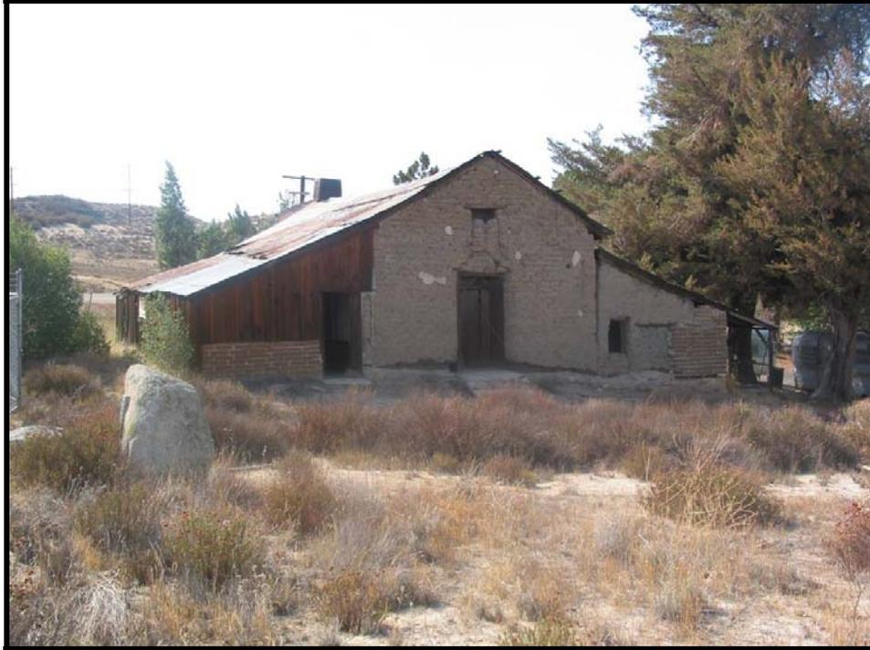
**Figure 26:** The east façade vividly illustrates the three different sections of the structure. The original two-room adobe can be seen in the center with the adobe addition to the north (right) and the wood/adobe addition to the south (left).
