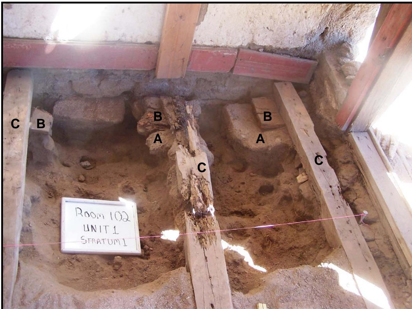
**Figure 61: Unit 10-1 excavated to 12 inches below surface. Note the large number of rodent burrows and the adobe blocks (A) supporting wooden boards (B), set under the floor sleepers (C).**
