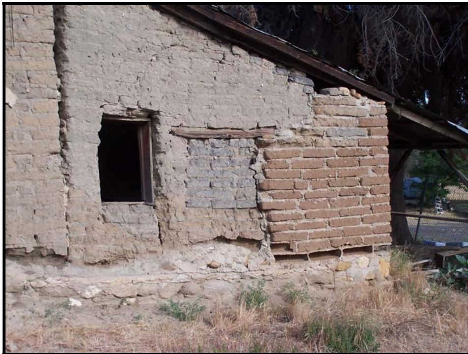
**Figure 27:** Multiple phases of construction can be seen in the east wall of the North Wing. Note how the wall is pulling away from the Central Wing on the left, suggesting a later period of construction.
