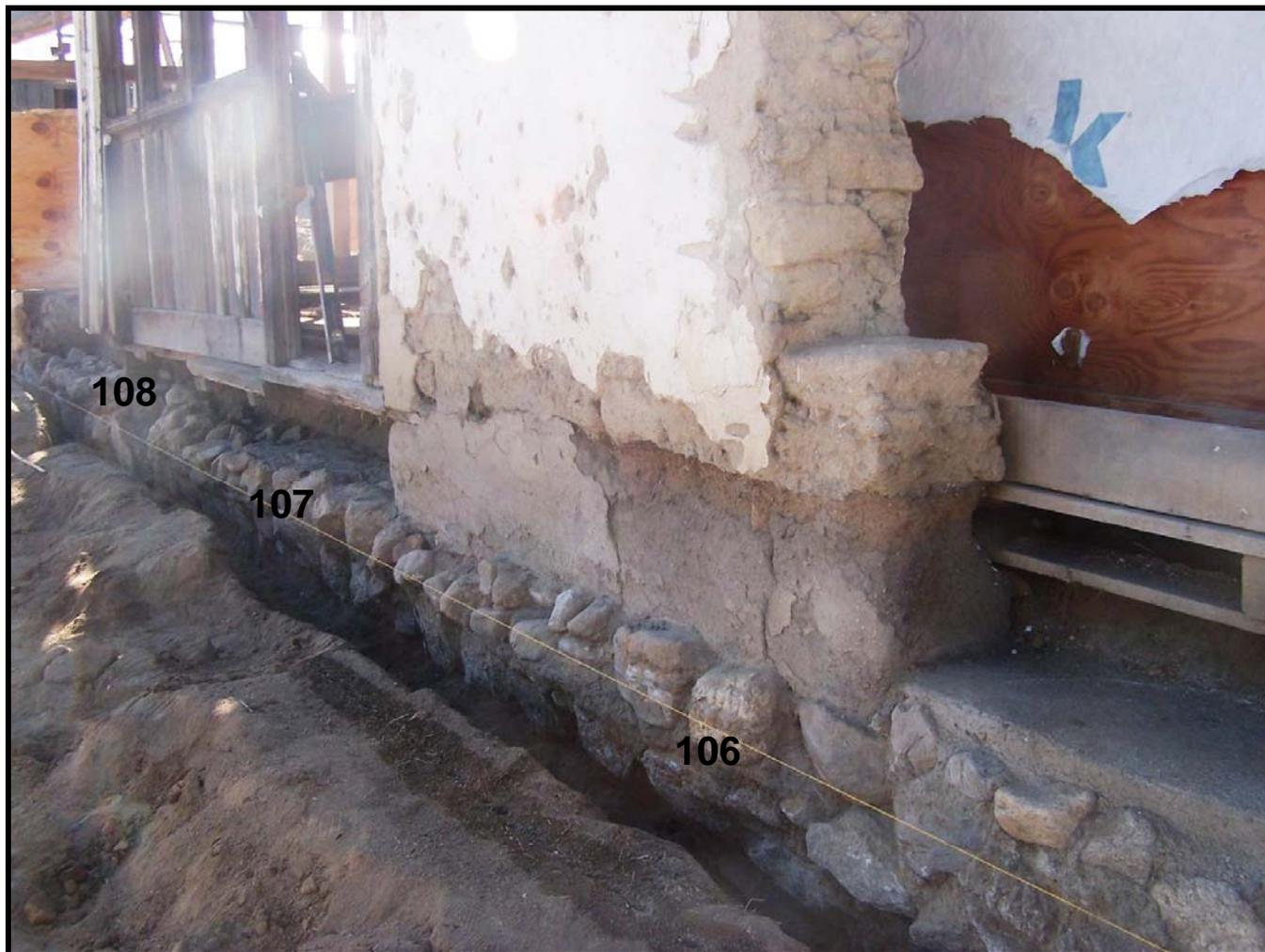
**Figure 76: North wall foundation of the North Wing exposed in the restoration construction trench along the northern edges of Rooms 106, 107 and 108. The segment at lower right was capped with concrete during stabilization activities in 2004.**
