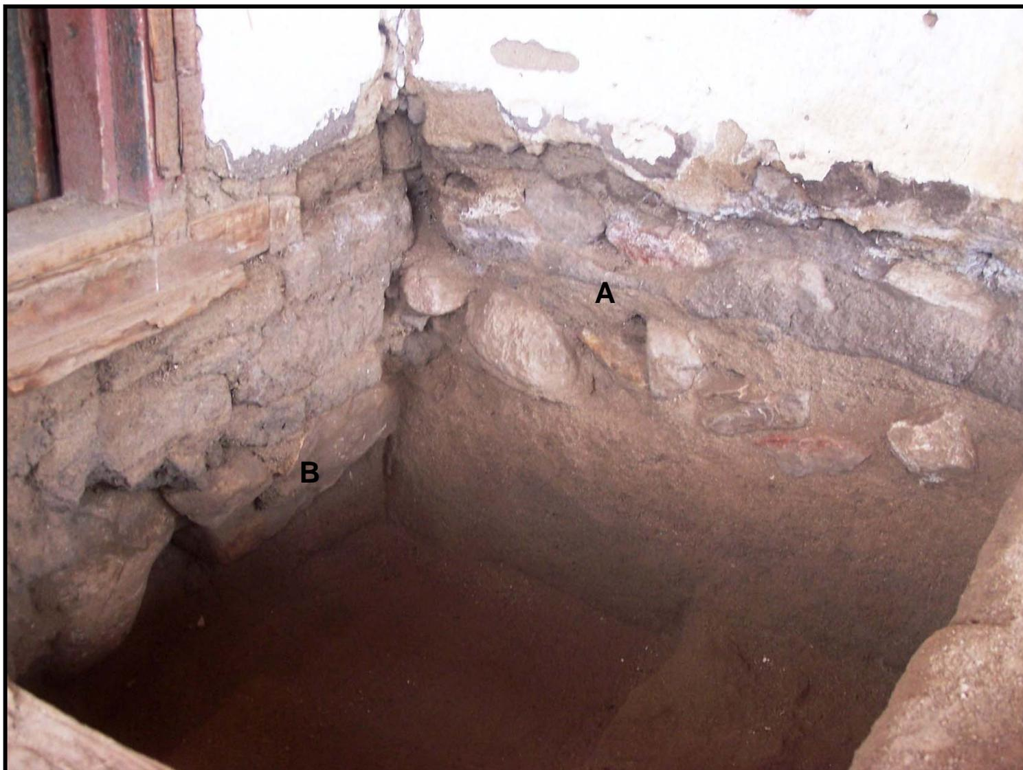
**Figure 59: Unit 3, Room 104, showing the west wall foundation of Room 103 (A) and the relationship between the angular granite field stone footing of the Central Wing (B).**
