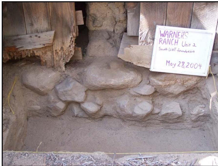
Figure 50: Cobble foundation and the end of the western interior dividing wall in Unit 04-2.
