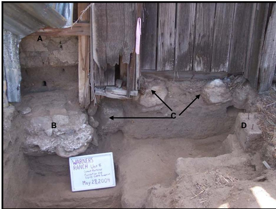
Figure 98: Unit 04-8, showing the adobe blocks of the west wall of the Central Wing (A), lime mortared cobble facing on the foundation of the Central Wing (B), and the remains of the cobble foundation for the original adobe wall on the west side of the South Wing (C), and wood support for the late 19<sup>th</sup> century addition (D).
