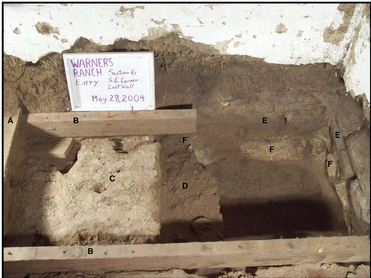
**Figure 38: Entry Room (101) block excavation Section 6 following excavation of the northeast corner, looking east. A portion of the far sleeper has been cut off to allow excavation access. Note (A) the present wooden floor board, (B) sleepers, (C) upper earthen floor, (D) lower earthen floor, (E) adobe blocks at the base of the wall, and (F) a single course of field stones underlying the wall.**
