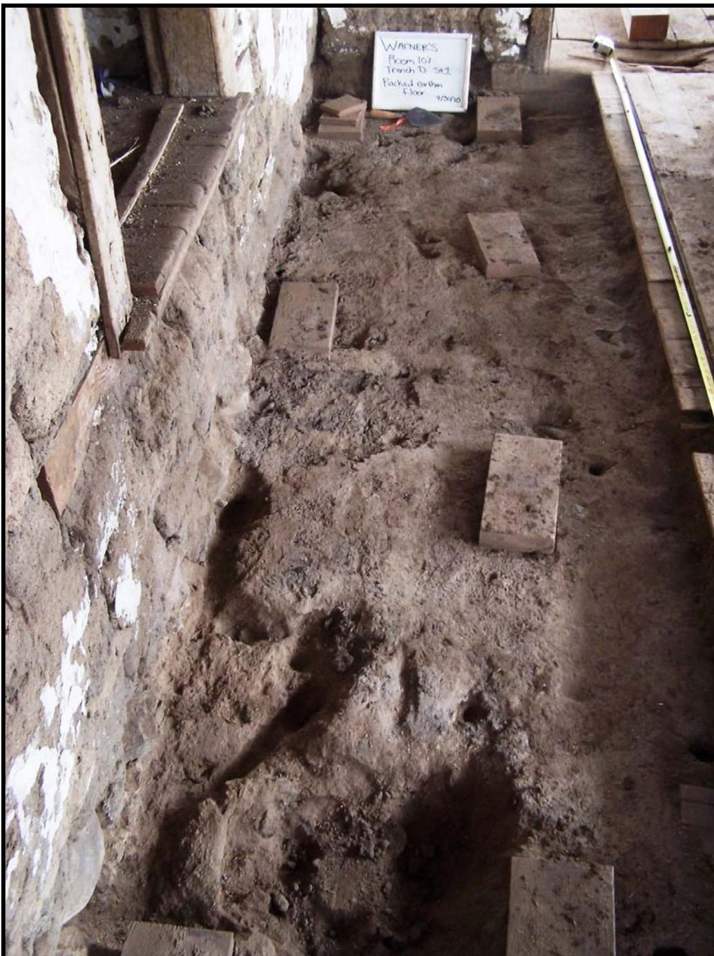
**Figure 80: Packed earthen floor uncovered in Trench D, Room 107, looking west. Once again note the boards placed on the surface to hold sleepers for the later wooden floors and the large holes caused by rodent burrowing.**
