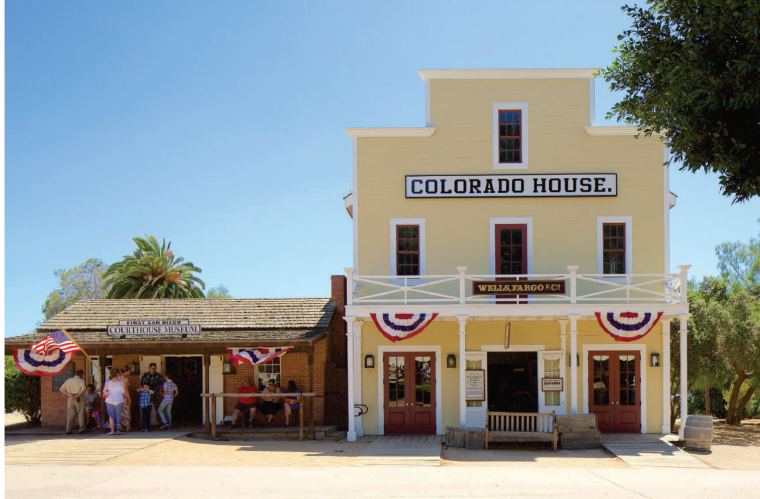
Reconstructed courthouse and Colorado House. 2024. Courtesy expedia.com
