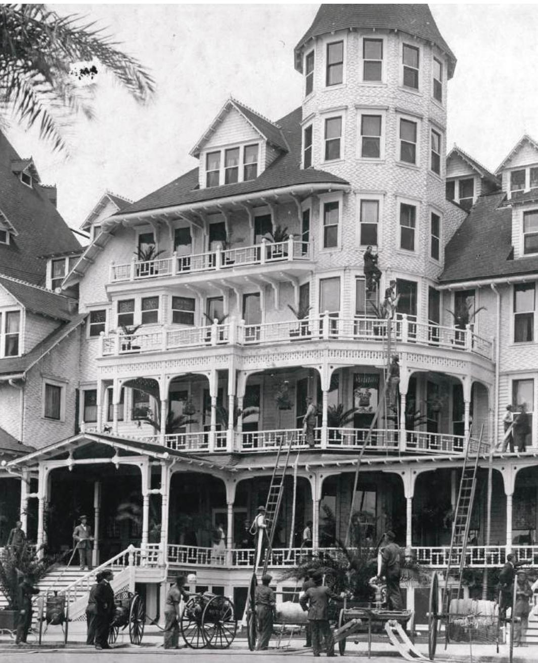
brackets and fretwork that once graced various areas from the first to fourth floors, were largely removed or replaced by the 1940s. The restoration has reinstated these Aesthetic Movement elements, blending their original historic charm with modern safety upgrades, such as adding frameless glass behind the railings to meet code.
