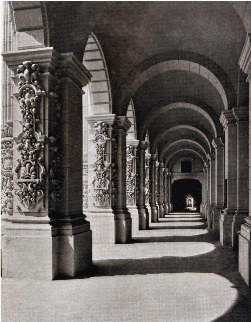
United States Building – the arcade.
