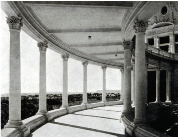
The Organ Pavilion peristyle.
