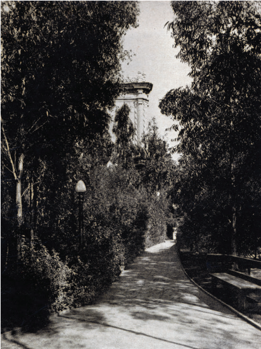
Commerce and Industries Building – portion of south façade.
