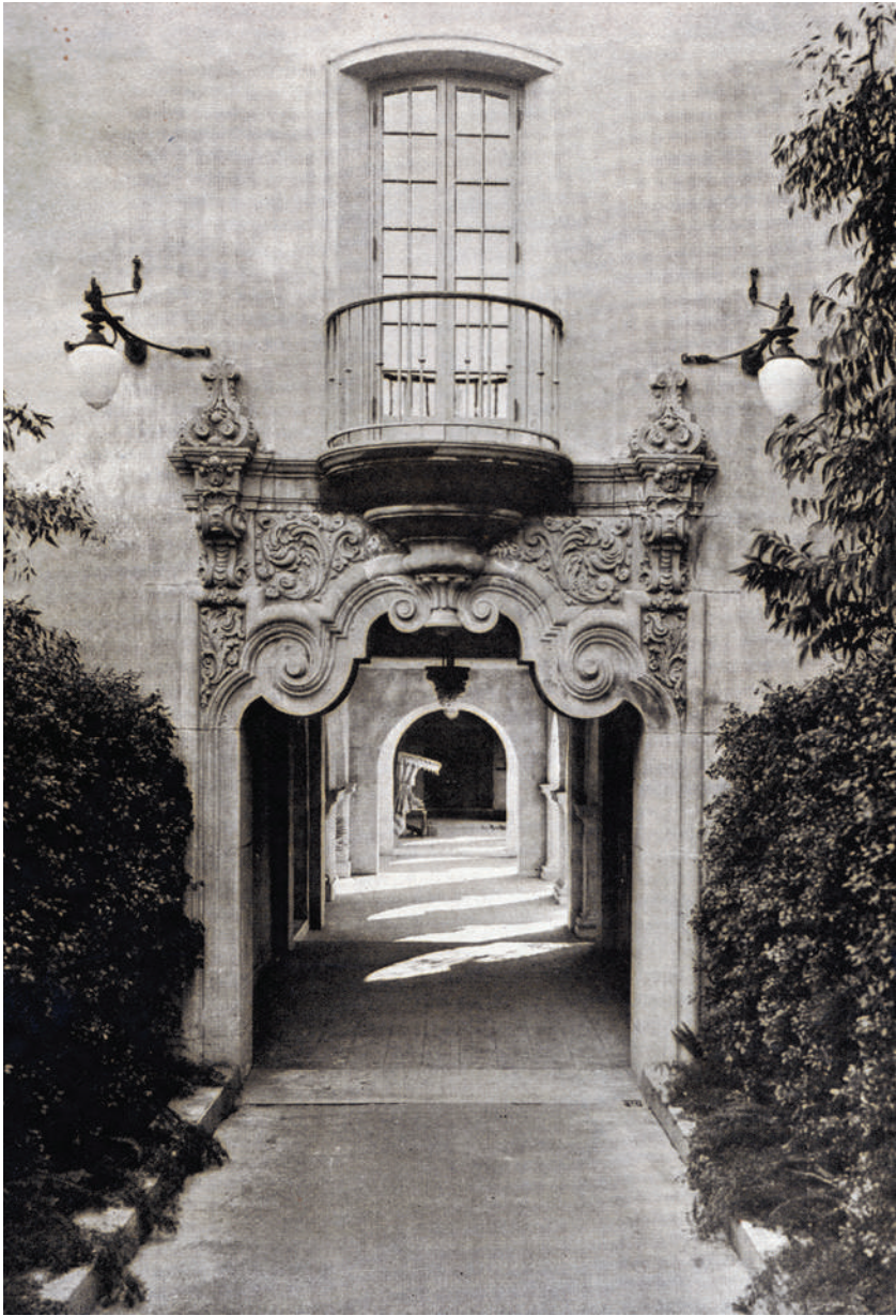
California Quadrangle – entrance from north gardens.
