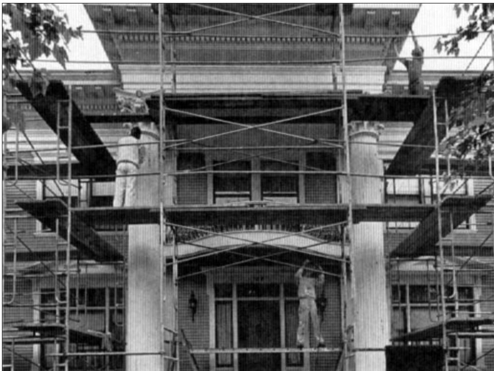
Ongoing work at this house focuses on the maintenance and repair of exterior wood features from the restoration period. After scraping and sanding, the wood was painted in colors documented to the Restoration period. Photo: ©Mary Randlett, 1992.
