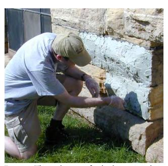
Figure 5. The application of a desalination poultice to a building is a technique used in architectural materials conservation. (Photo by author.)
