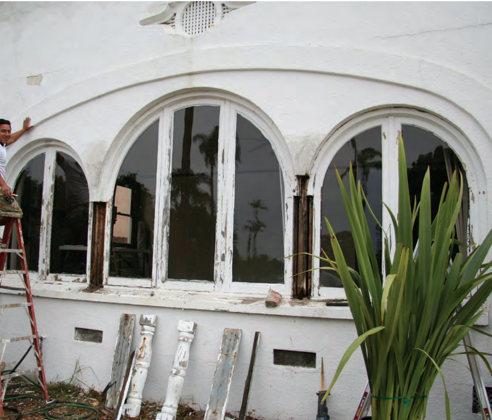
Current restoration of a 1921 Morris Irvin Spanish Revival home, workmen are restoring decorative pilasters.
