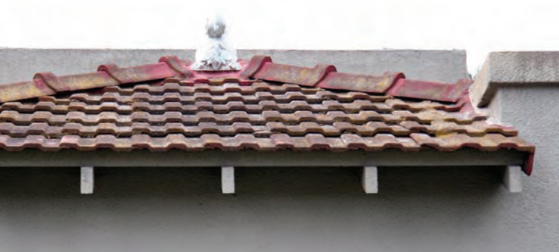
Above Roman tiles on a 1920 Morris Irvin Mission Revival home and exposed rafter tails; right Original Roman tiles on another Morris Irvin Mission Revival home with diminutive bell tower and decorative balcony. A sensitive addition lies toward the back of this 1921 home.
