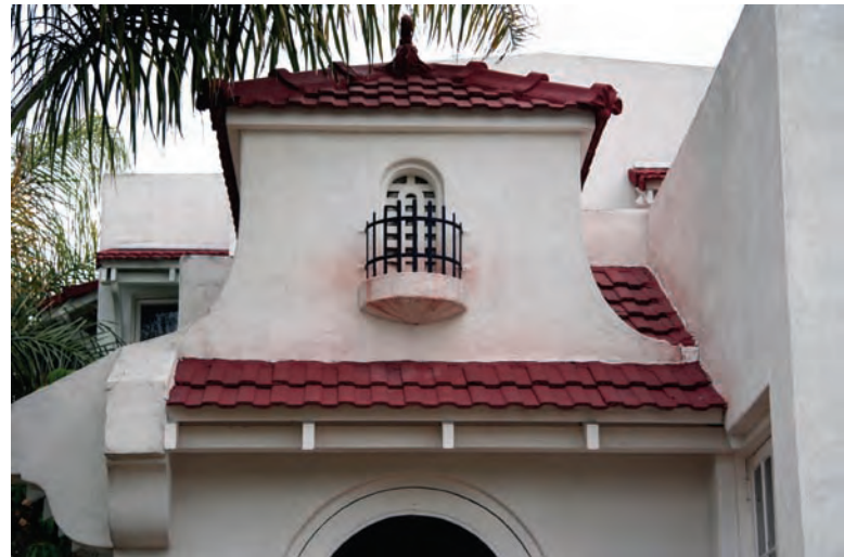
Above Roman tiles on a 1920 Morris Irvin Mission Revival home and exposed rafter tails; right Original Roman tiles on another Morris Irvin Mission Revival home with diminutive bell tower and decorative balcony. A sensitive addition lies toward the back of this 1921 home.
