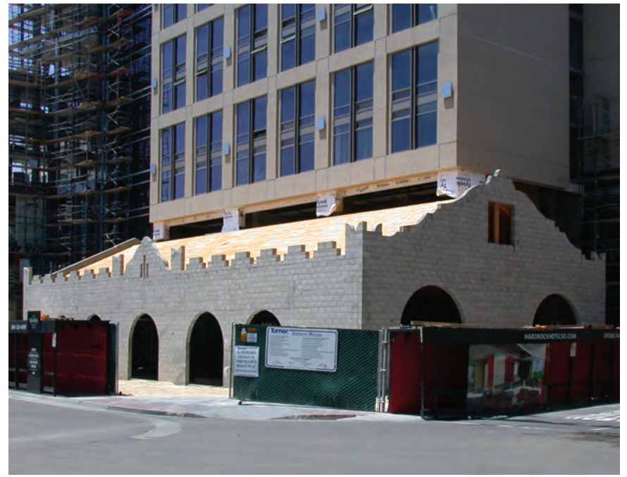
above National City & Otay Depot under reconstruction, 6th Avenue and K Street, awaiting installation of its original brick, the application of stucco, tin roof, and star window, photo Bruce Coons; below Elevations of the NC&O reconstructed building, 2006, left south side; right east side, courtesy of Heritage Architecture and the Hard Rock Hotel.
