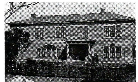
The 1894 Grant House was designed to face downtown; the current "front" on 6th & Quince is actually the back of the house. This view is the real front, now hidden in the backyard.
