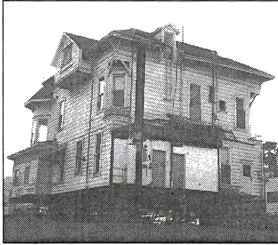
The Ginty House may now have a low foundation, but it doesn't have a restoration.
