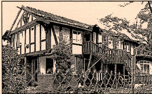
'The partially demolished Barber House.
