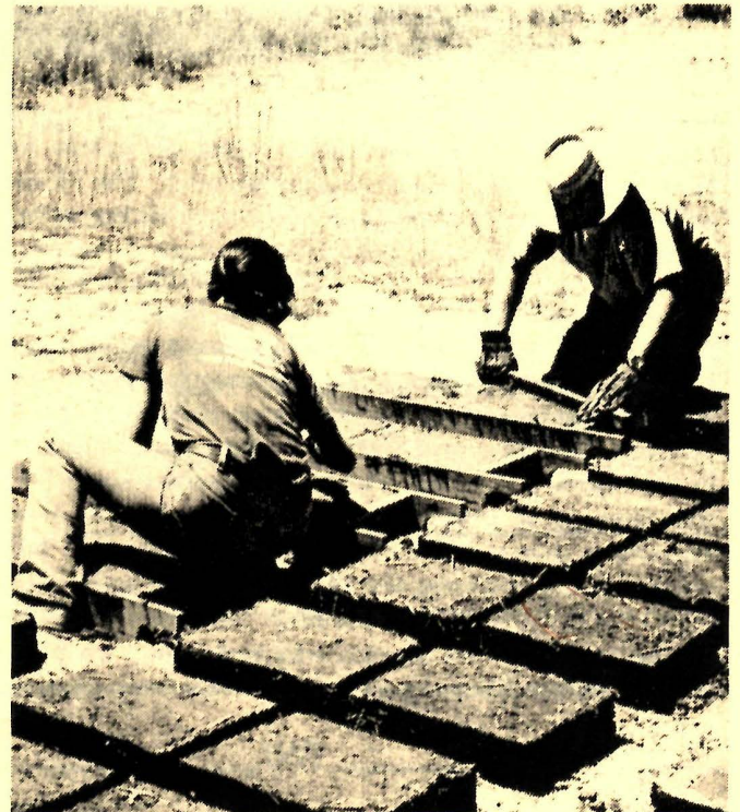
Adobe making at St. Francis Chapel
