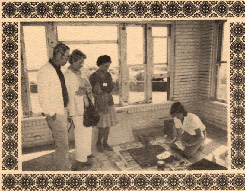
Tina Hallen demonstrates floor laying
