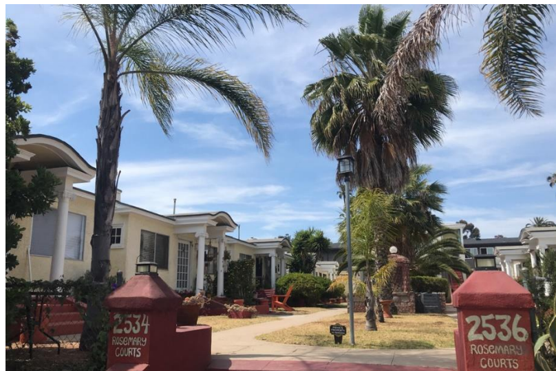
Figure 6. 2538 B Street, an early bungalow court constructed in 1921 in Golden Hill.
