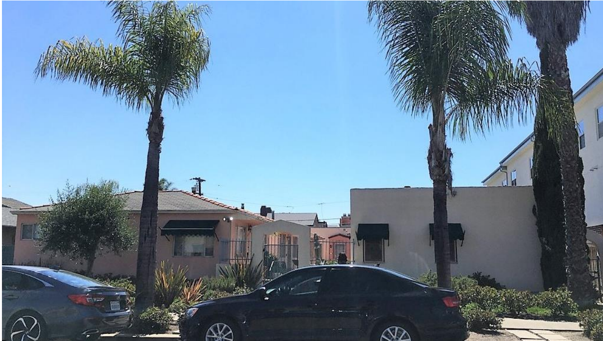
Figure 24. Hybrid bungalow court with Pubelo-style units constructed in the 1920s or 1930s (right) and Minimal Traditional units constructed in the 1950s (left).
