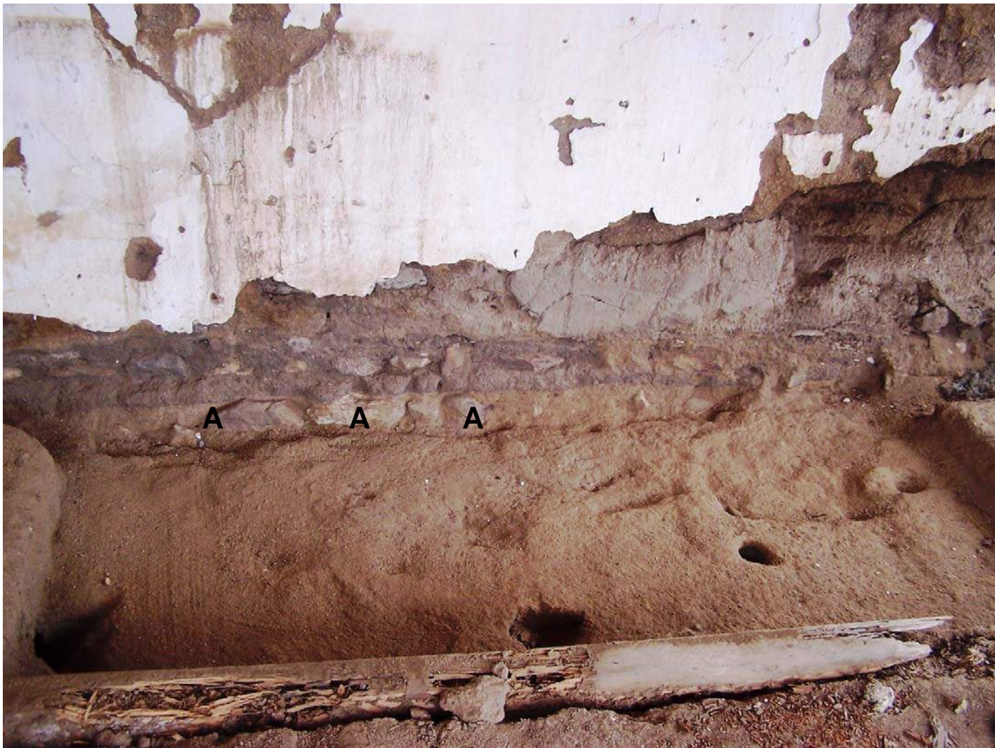
Figure 70: Compact surface uncovered in Trench B, Room 104, looking toward the east wall of the room. Note how the foundation cobbles (A) appear to have been laid upon this surface.
