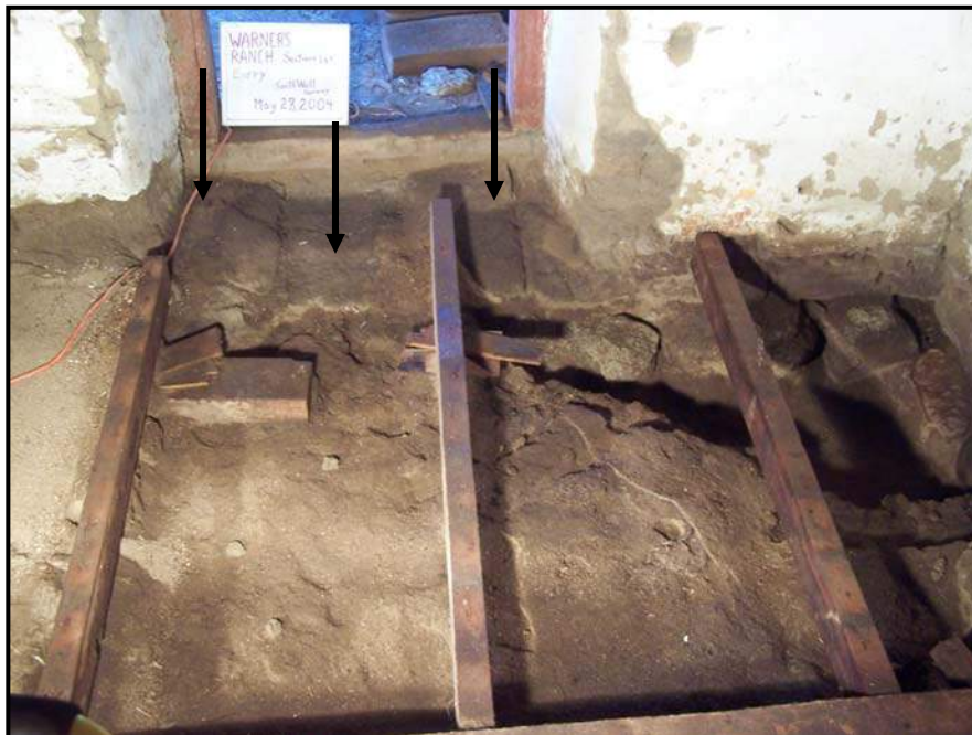
Figure 42: Entry Room (101) Block excavation Sections 2 and 3. The badly worn lower earthen floor and blocks in the door way can clearly be seen.
