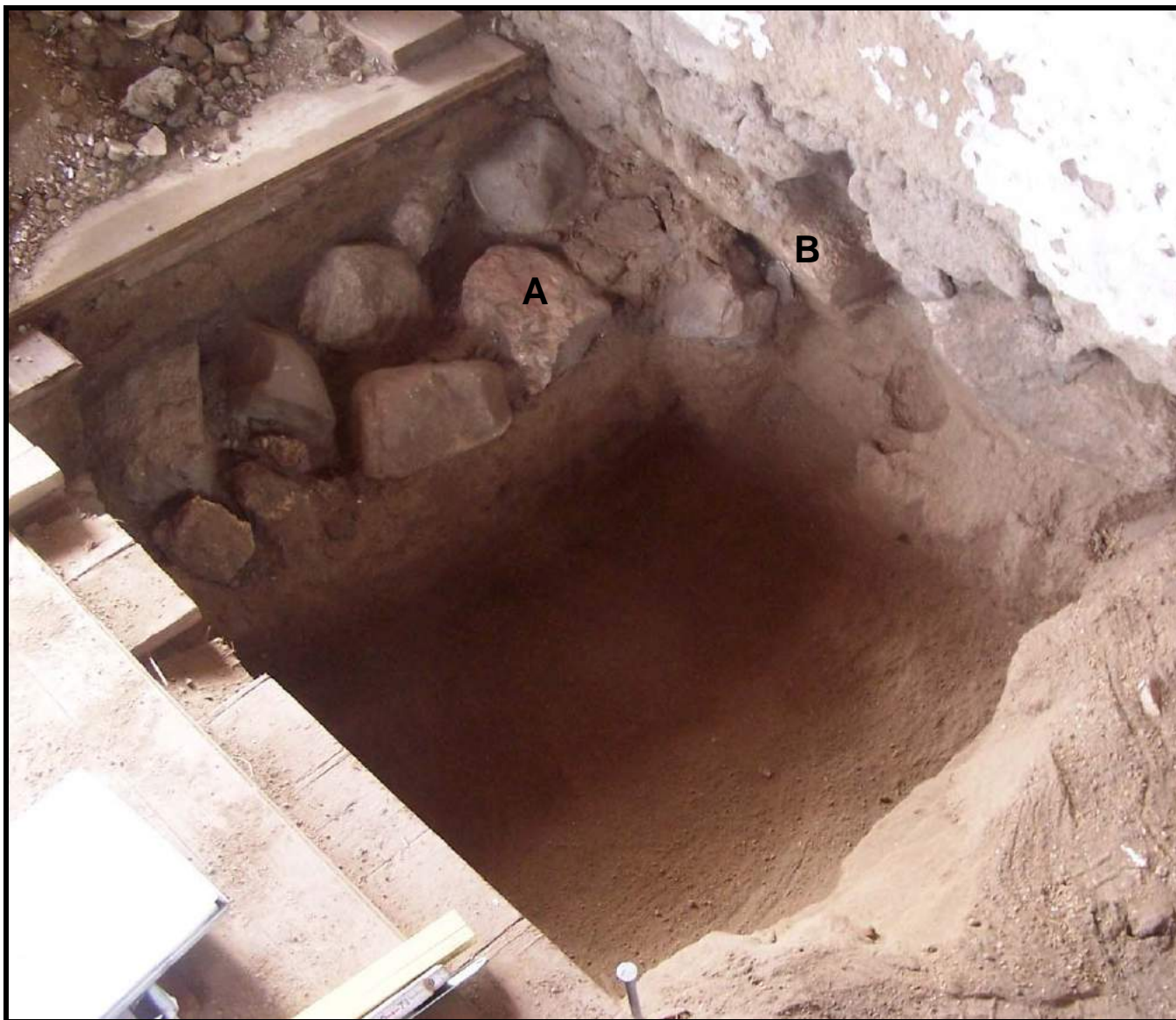
Figure 83: The single course cobble foundation for the dividing wall between Rooms 107 and 108 (A) built against the irregular granite field stone footing of the north wall of Room 105 (B).
