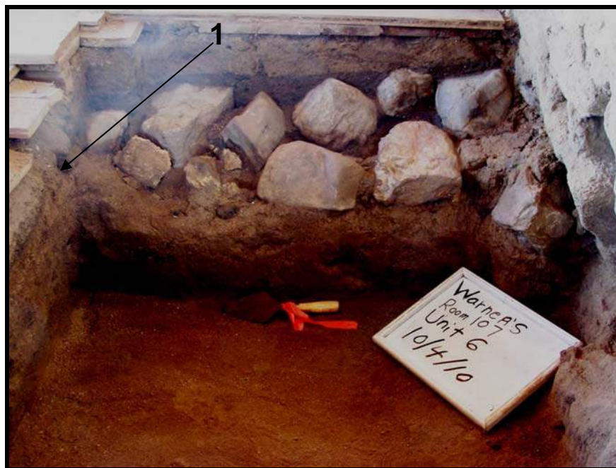
Figure 82: Interior dividing wall foundation between Rooms 107 and 108 as seen in the east sidewall of Unit 10-5 in Room 107. The dark brown band is the mud mortar in the south side wall profile shown above. Point 1 is the same location in both figures and shows the contact between the wall mortar and the earthen floor. The Photo ID Board is incorrectly labeled Unit 6.
