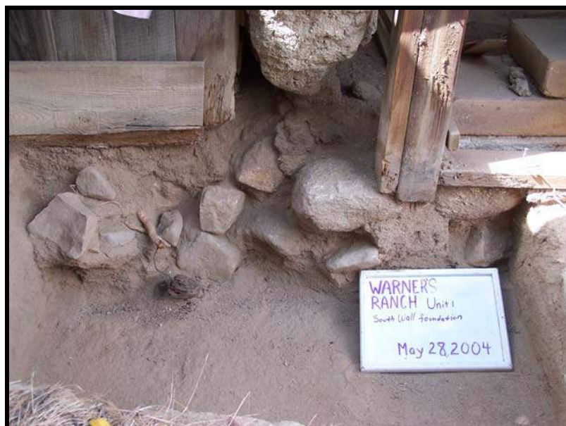
Figure 54: Cobble foundation in Unit 04-1. The west half (left) is badly disturbed while the eastern portion remains intact.
