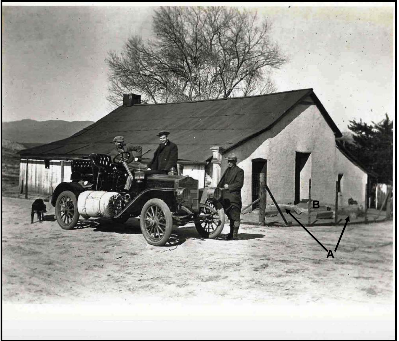
Figure 13: The Ranch House about 1910. The picket fence is gone. Note the board and batten siding on the south side behind the car, the sheet metal roof, the well maintained white wash exterior, the stone facing along the base of the east side (A) and the concrete mortared stone steps (B) (Courtesy San Diego History Center).
