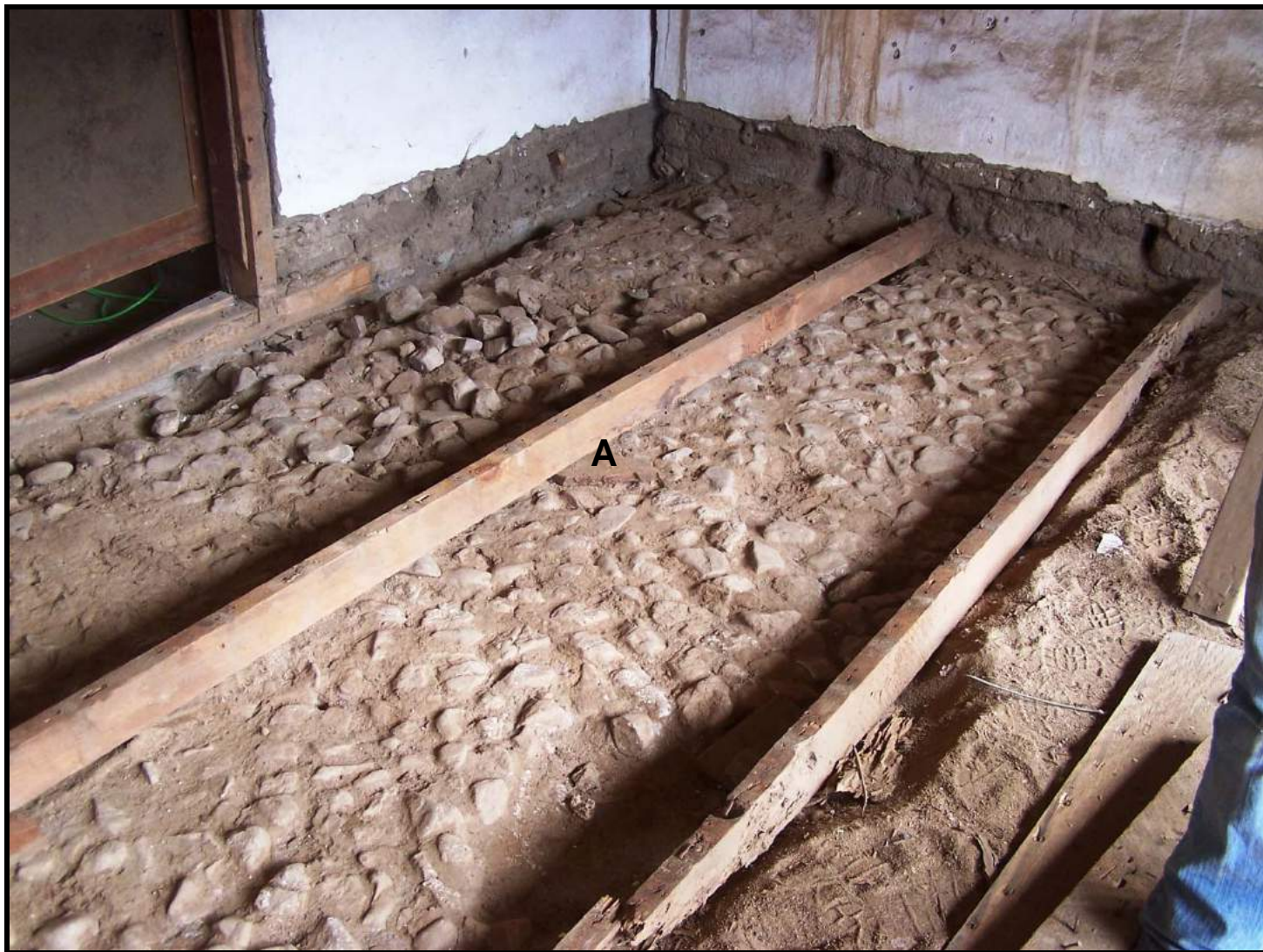
Figure 66: Another view of the cobble floor uncovered in Room 103, looking toward the northeast corner. "A" marks the same reference point as in Figures 64 and 65.
