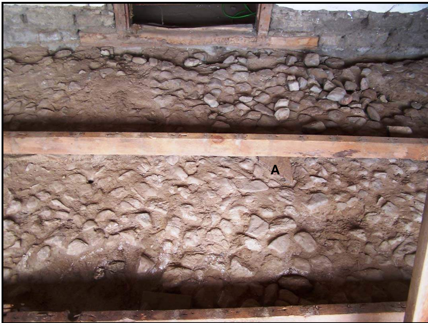
Figure 65: Center portion of the cobble floor uncovered in the north half of Room 103, looking toward the north wall. "A" marks the same reference point as in Figures 64 and 66.
