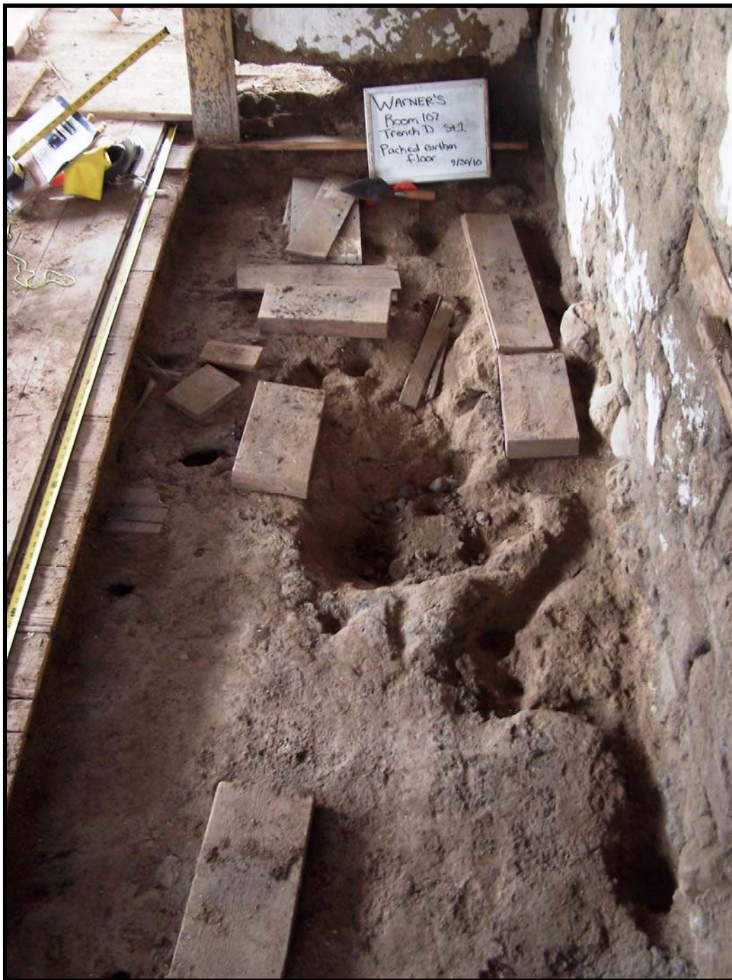
Figure 79: Packed earthen floor uncovered in Trench D, Room 107, looking east. Note the boards placed on the surface to hold sleepers for the later wooden floors and the large holes caused by rodent burrowing.
