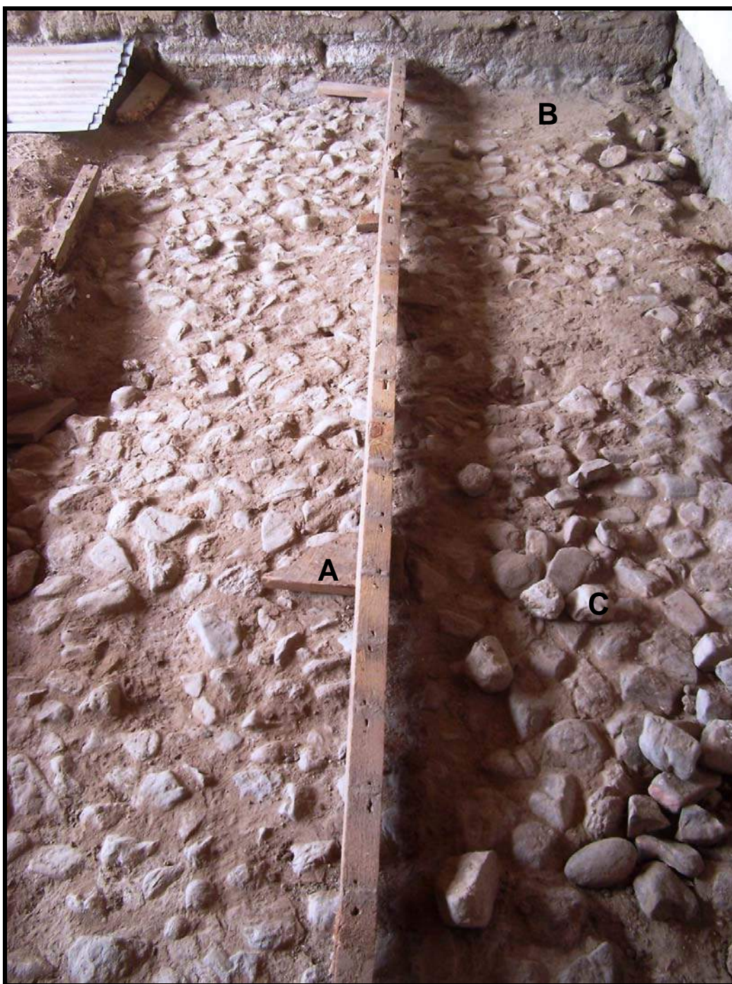
Figure 64: Densely packed cobble floor in the north half of Room 103, looking toward the west wall. The board (A) beneath the 2 by 4 inch sleeper will be referenced in the following two photographs. Note the intact surface where the mud grout still covers the cobbles in the northwest corner (B), and the loose cobbles in the right foreground (C).
