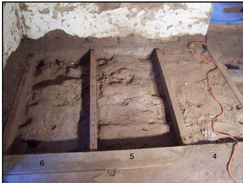
Figure 36: Sections 4, 5, and 6 of the Entry Room (101) block excavation showing the upper packed earthen floor surface that was exposed after the loose fill between the sleepers was removed. The fill has not been taken out in Section 4.
