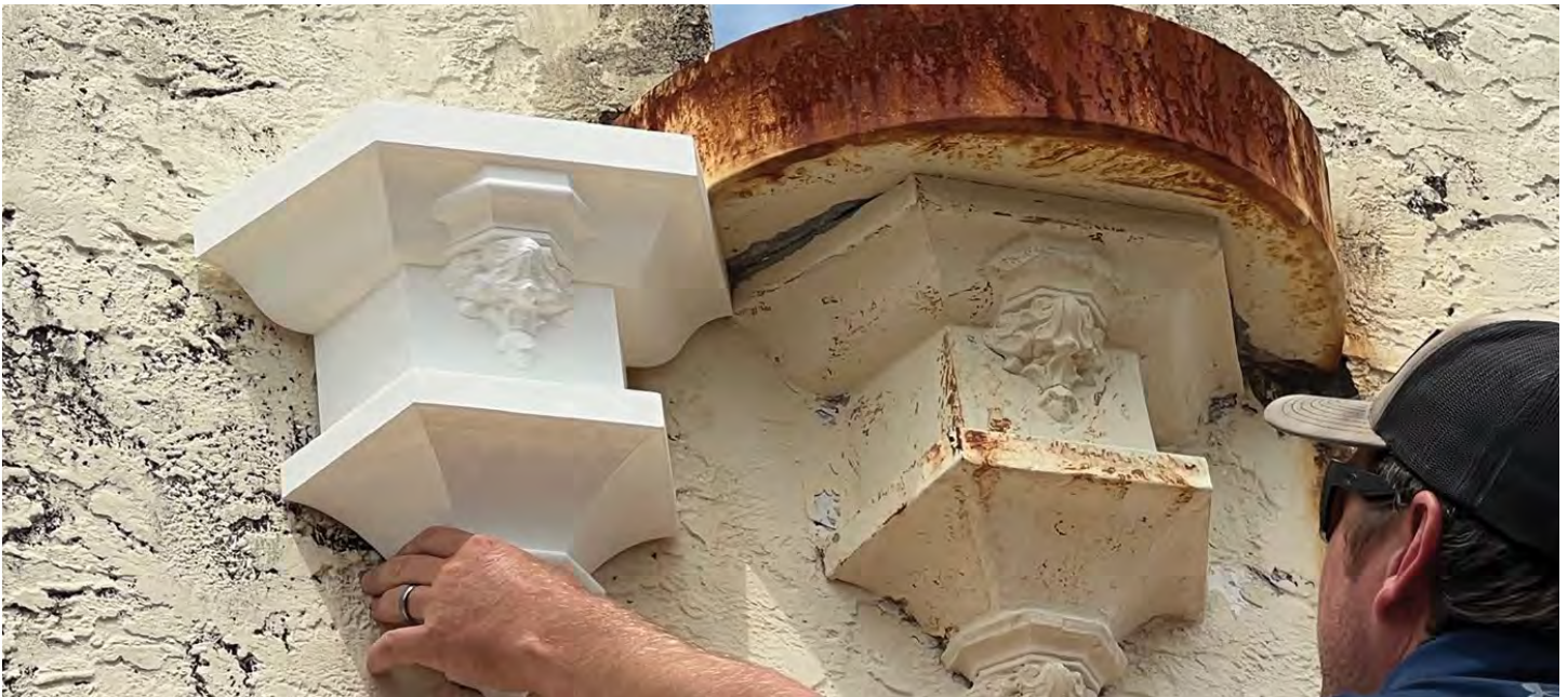
Figure 23. 3-D printing using various polymers is occasionally used to replicate missing metal or wood features. This new application is continually being refined, but the application can be successful when a painted, lightweight feature needs to be replicated. Photo: NPS.
