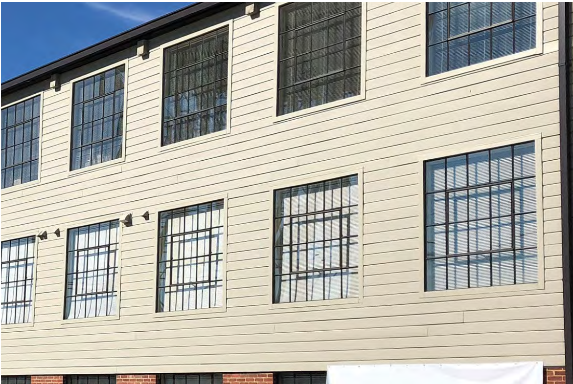
Figure 21. A mineral polymer composite siding was available in the profile very similar to the historic siding. The replacement siding was used where the original material was almost completely missing beneath a more modern covering. Areas where the original wood were largely intact were replaced with matching wood to sustain more of the material integrity of the building. Photo: Belk Architecture.
