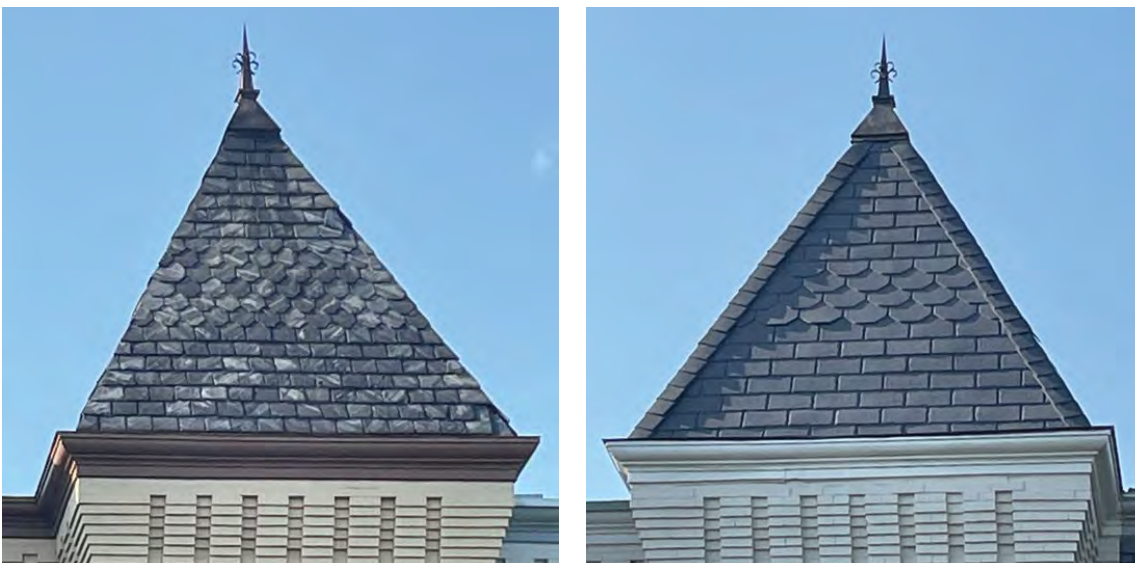
Figure 10a and 10b. Polymer slates offer a choice of shapes but not sizes, limiting their ability to achieve a good visual match for some historic slate. With the size of the polymer slates (Figure 11b) being nearly twice that of the historic slates (11a), the scale of the entire feature is incompatibly altered. The molded edges of this material, which contribute to its ability to replicate slate, would be lost if each shingle was resized by cutting. Photo: John Sandor, NPS.
