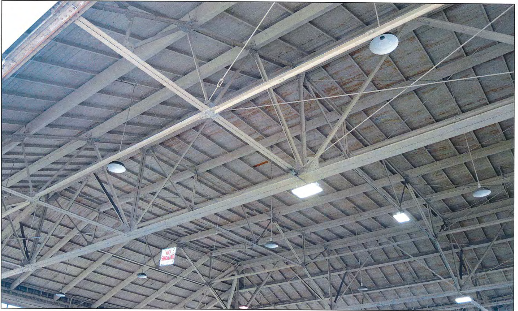
Plate 3.3.7-5 View of the Wood Plank Ceiling of the UAHT Building, Facing Southeast The SDIA Airport Development Plan Project
