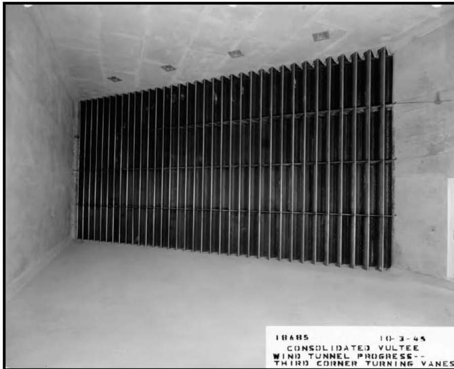
Plate 3.3.9-7: CWT building turning vanes in 1945. (Photograph courtesy of the San Diego Air and Space Museum)
