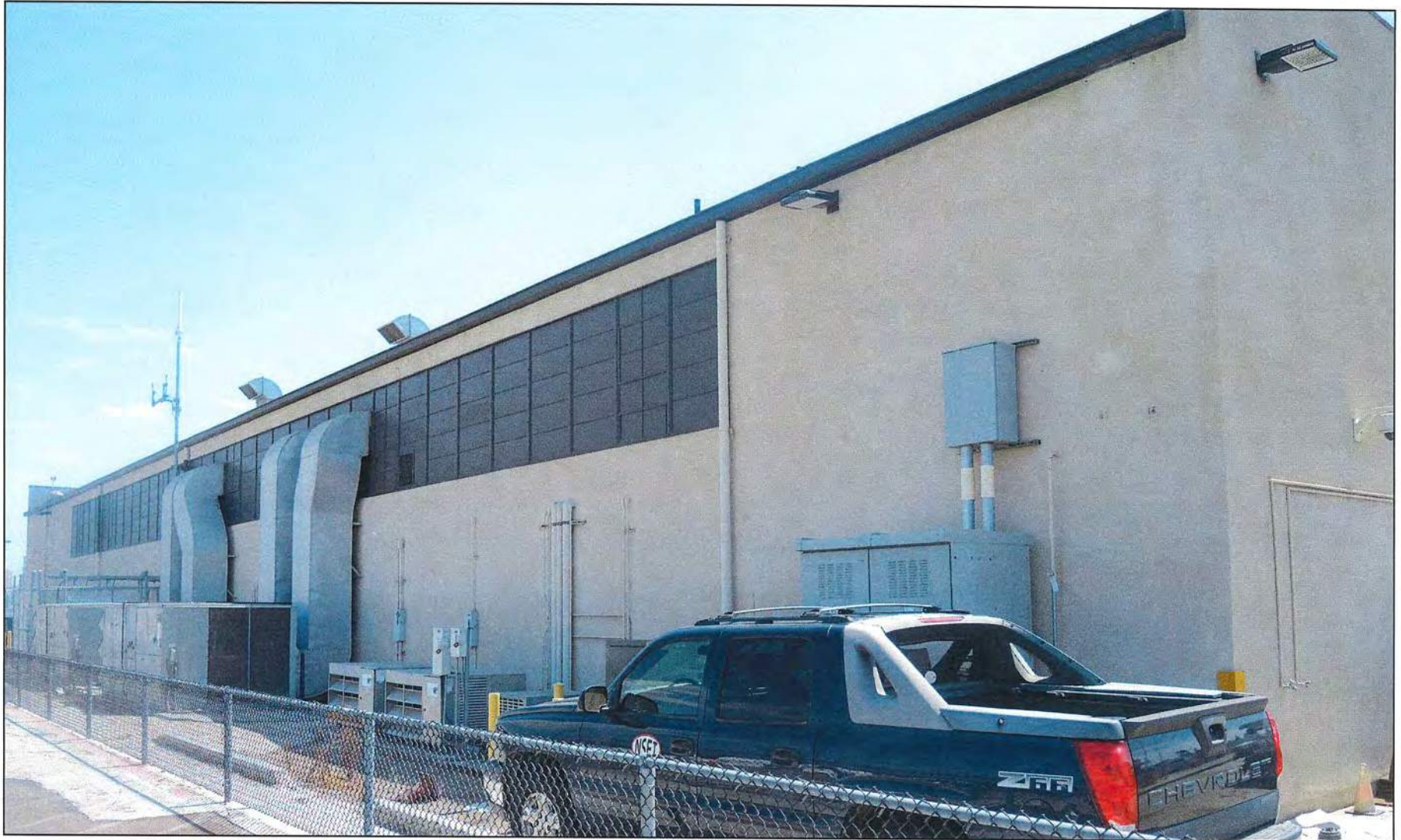
Plate 3.3.8-6 View of the North Façade of the JEO Building Showing the Horizontal Band of Steel-Framed Windows, Facing Southeast The SDIA Airport Development Plan Project
