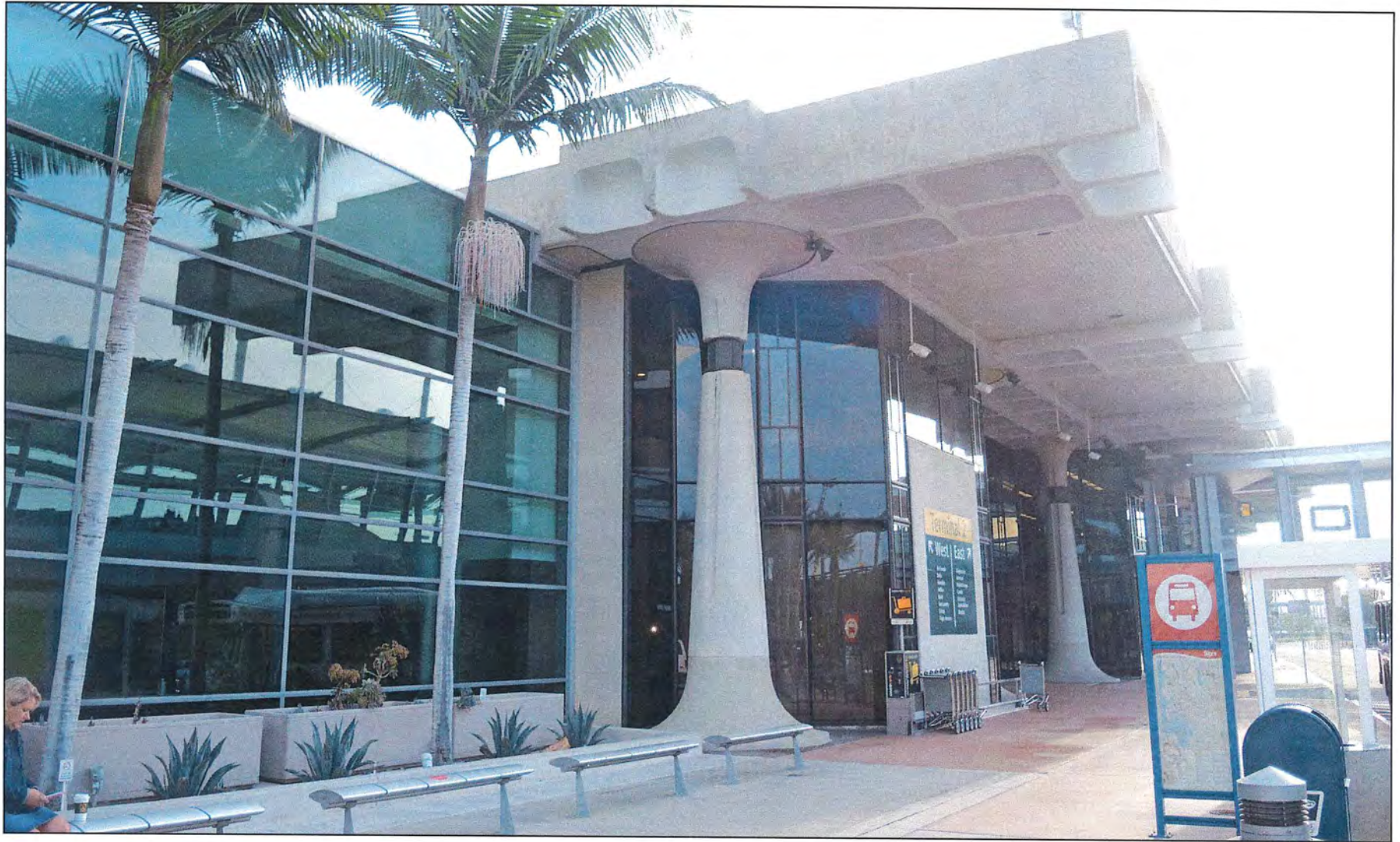
Plate 3.3.2-10 View of the Coffered Concrete Overhang and a Concrete Support Column on the West Façade of Section A, Facing Northeast
