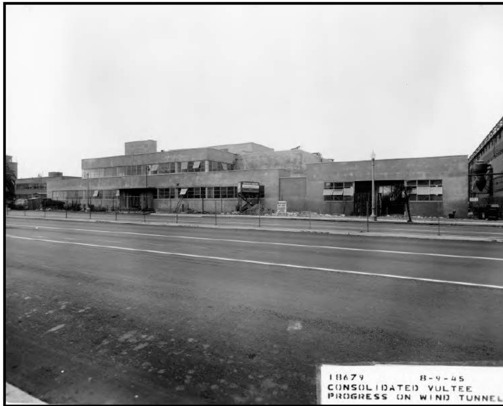
Plate 3.3.9–1: View of the CWT building under construction in 1945. (Photograph courtesy of the San Diego Air and Space Museum)
