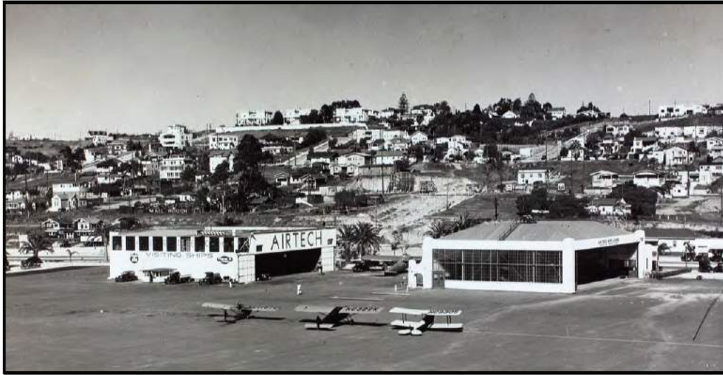
Plate 1.2–3: Airtech hangar and the Pacific Air Transport/United Airlines Terminal circa 1931 to 1932. (Photograph courtesy of the San Diego Air and Space Museum)
