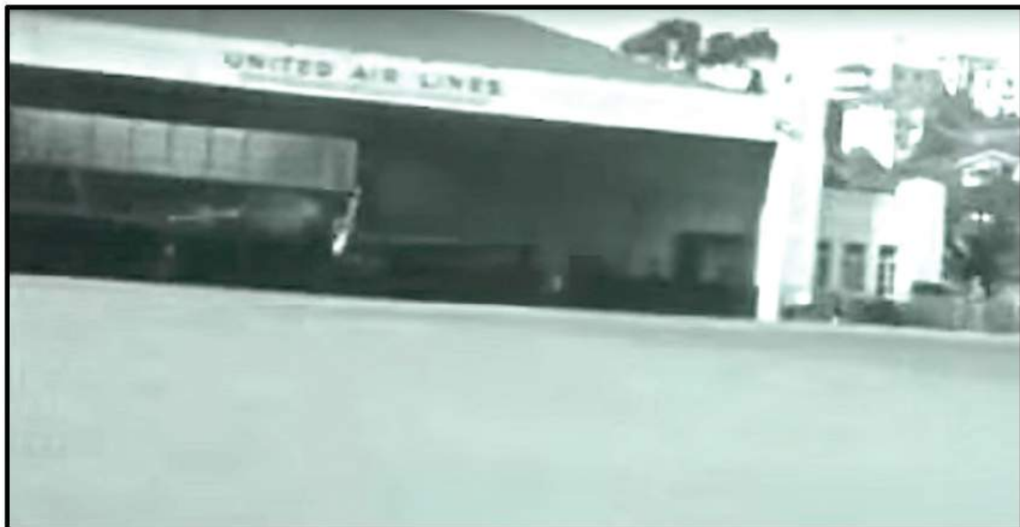
Plate 3.3.7-14: Circa 1931 to 1941 photograph of the interior of the UAHT building showing the attached terminal and two entrance doors on the right side. (Photograph courtesy of the San Diego Air and Space Museum)
