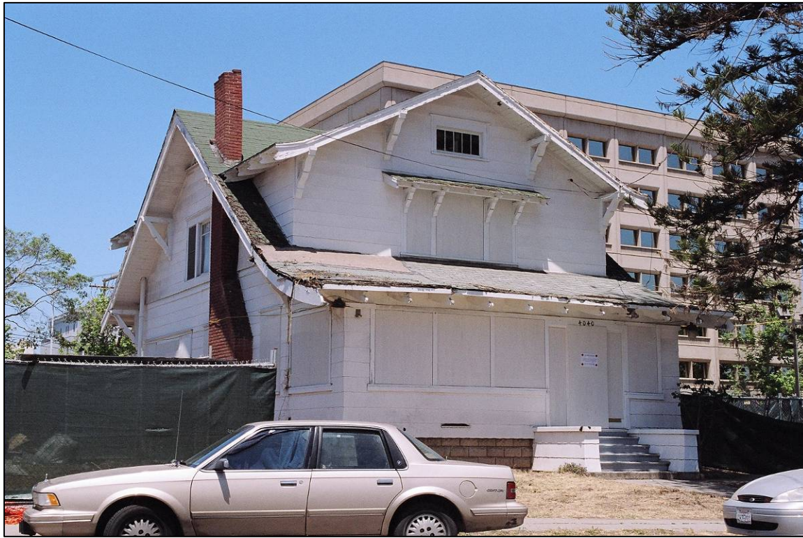
Photograph 1 Overview of House
