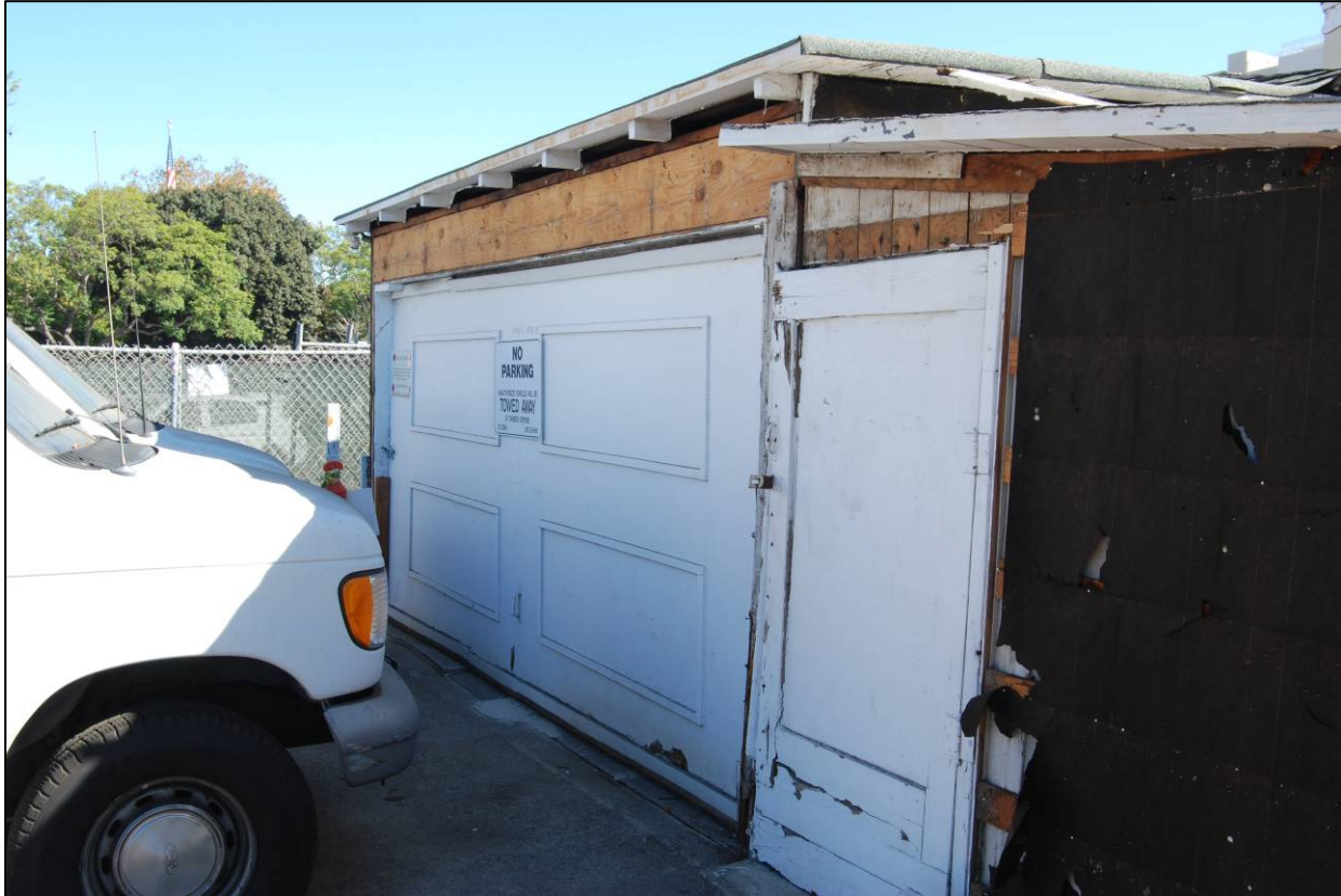
Photograph 32 West Side of Garage Showing Both West Addition and South Addition.
