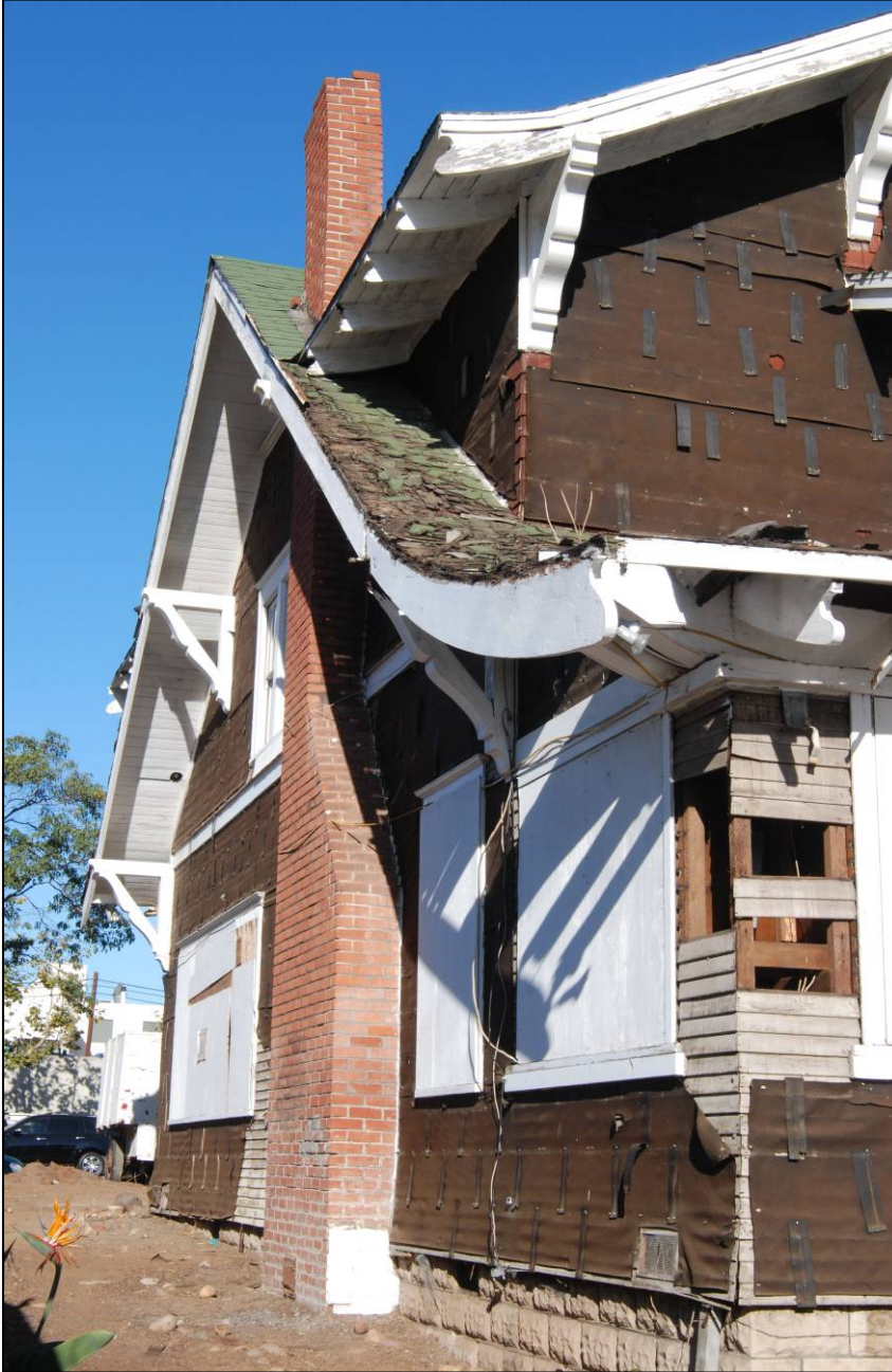
Photograph 24 Chimney on South Side
