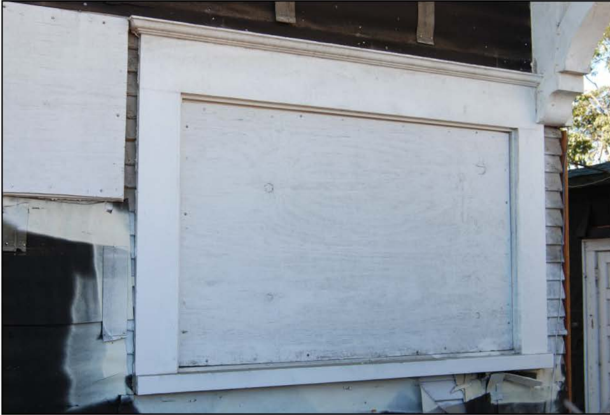
Photograph 14 Casing on Windows on Main Portion of House. Note wide side and top casing boards and decorative trim at top.
