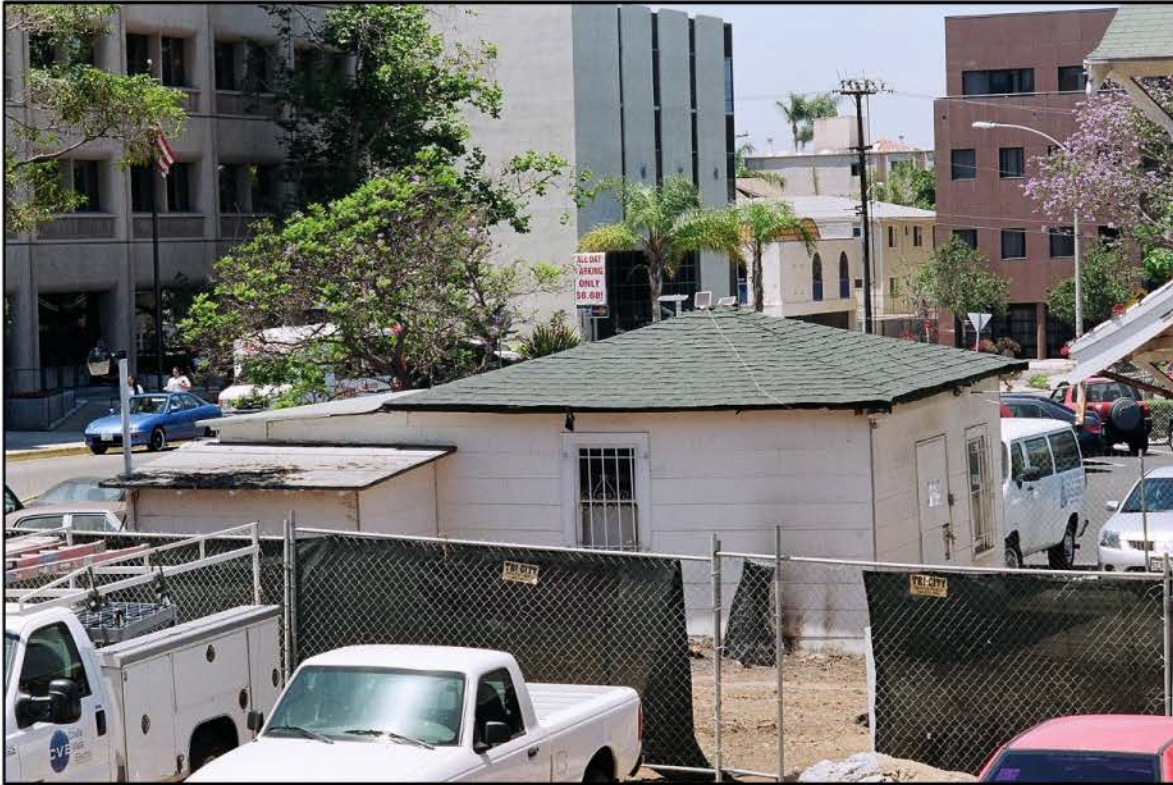
Photograph 28 Overview of Garage Building, Taken Before Siding Was Removed
