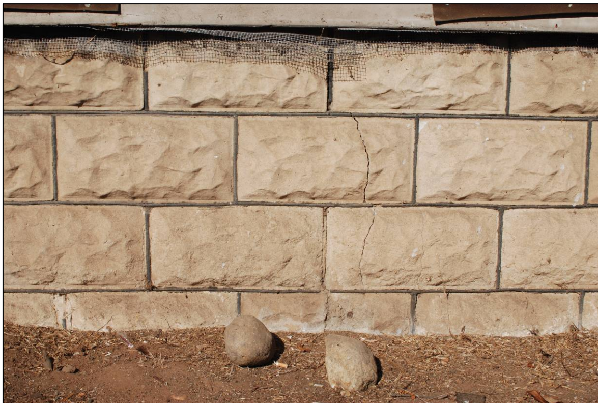
Photograph 2 Foundation, Concrete Block Formed to Resemble Dressed Stone
