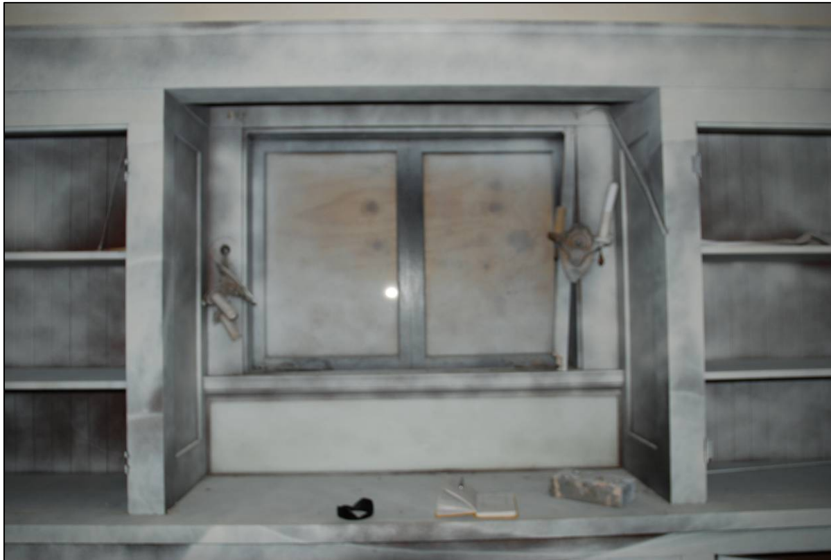
Photograph 26 West Side, South Window, Interior Shot
