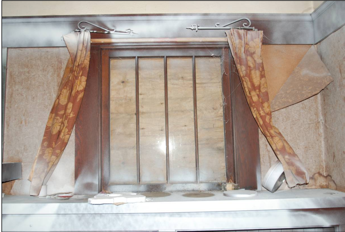
Photograph 21 Southe Side Window 2, Interior Shot.
