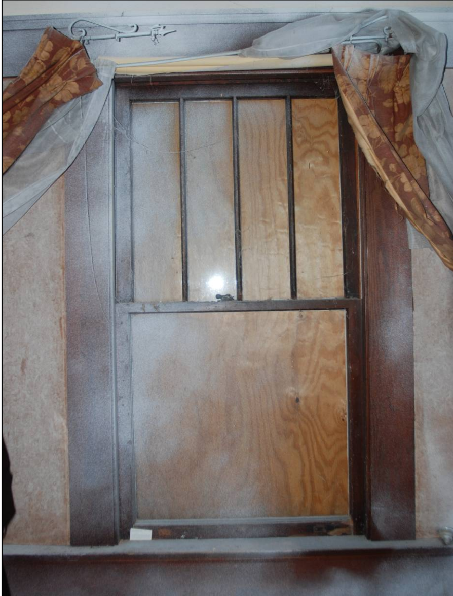
Photograph 20 South Side Window 1, Interior Shot
