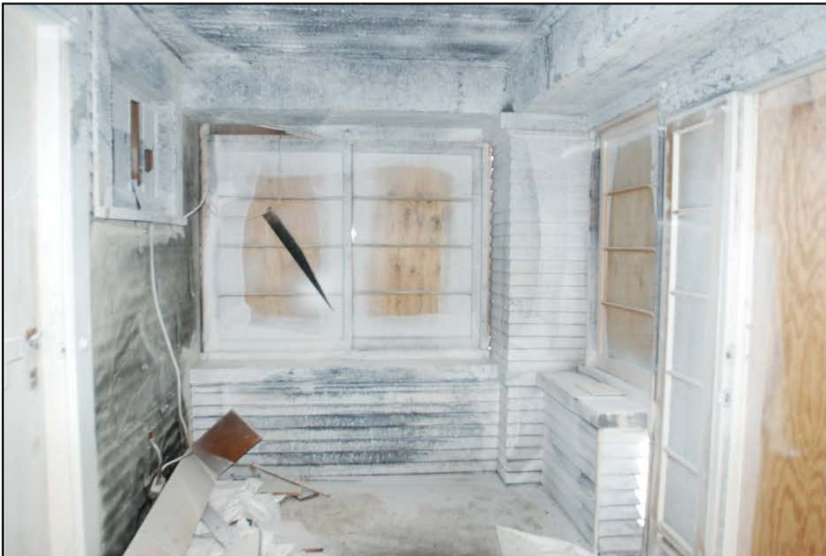
Photograph 10 Interior of Porch, Looking North
