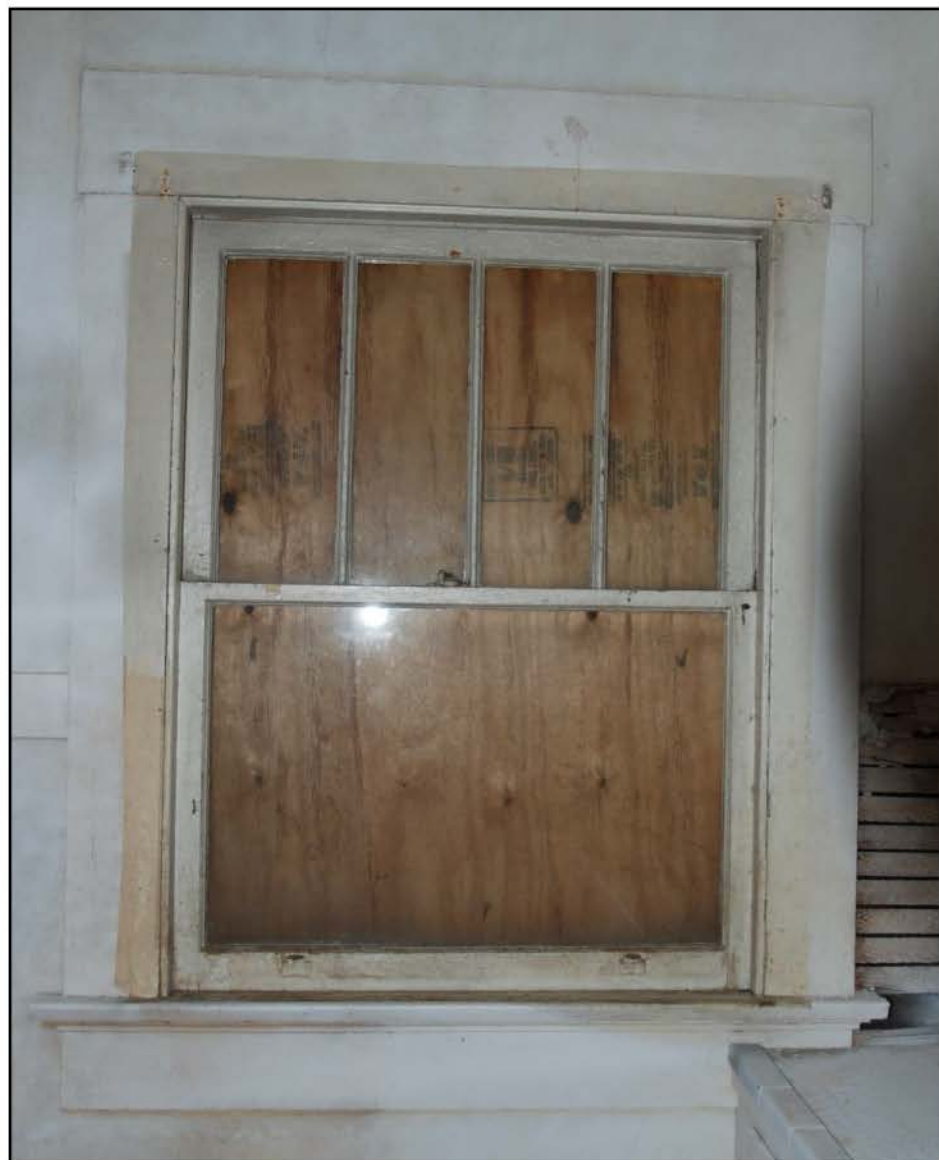
Photograph 16 North Side Window 3, Interior shot.
