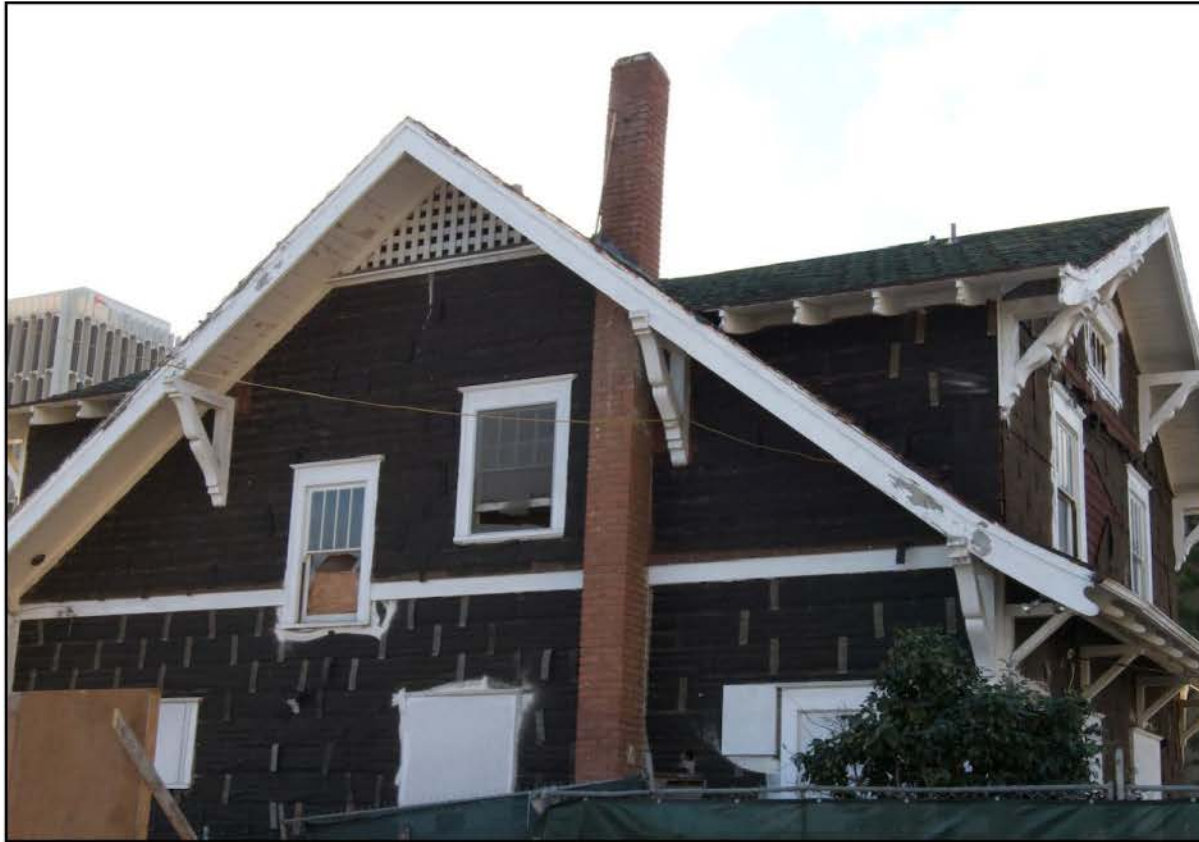
Photograph 18 Northeast Corner of House, Showing Small Chimney on North Wall
