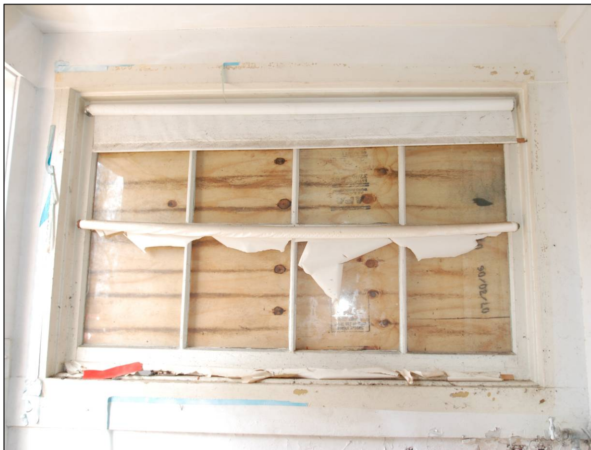
Photogrtaph 17 Window 4, Interior Shot
