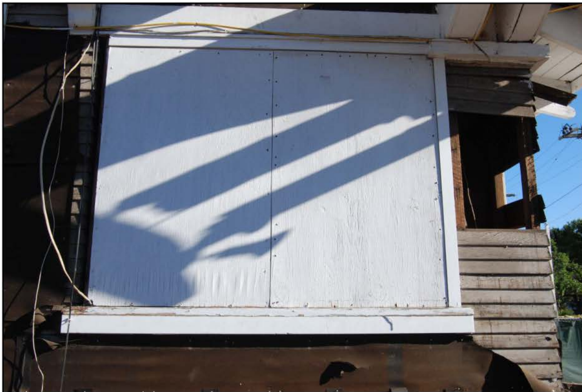
Photograph 8 Window Casing Detail on Front Porch Windows, Note Narrow Side and Top Casing Boards. This is South Side Window
