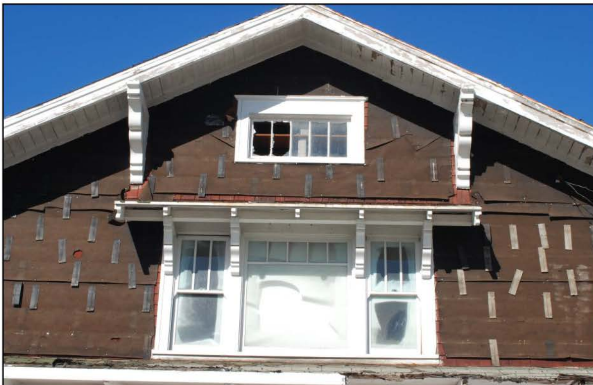
Photograph 13 Second Floor and Attic Windows on West Side (Front) of House
