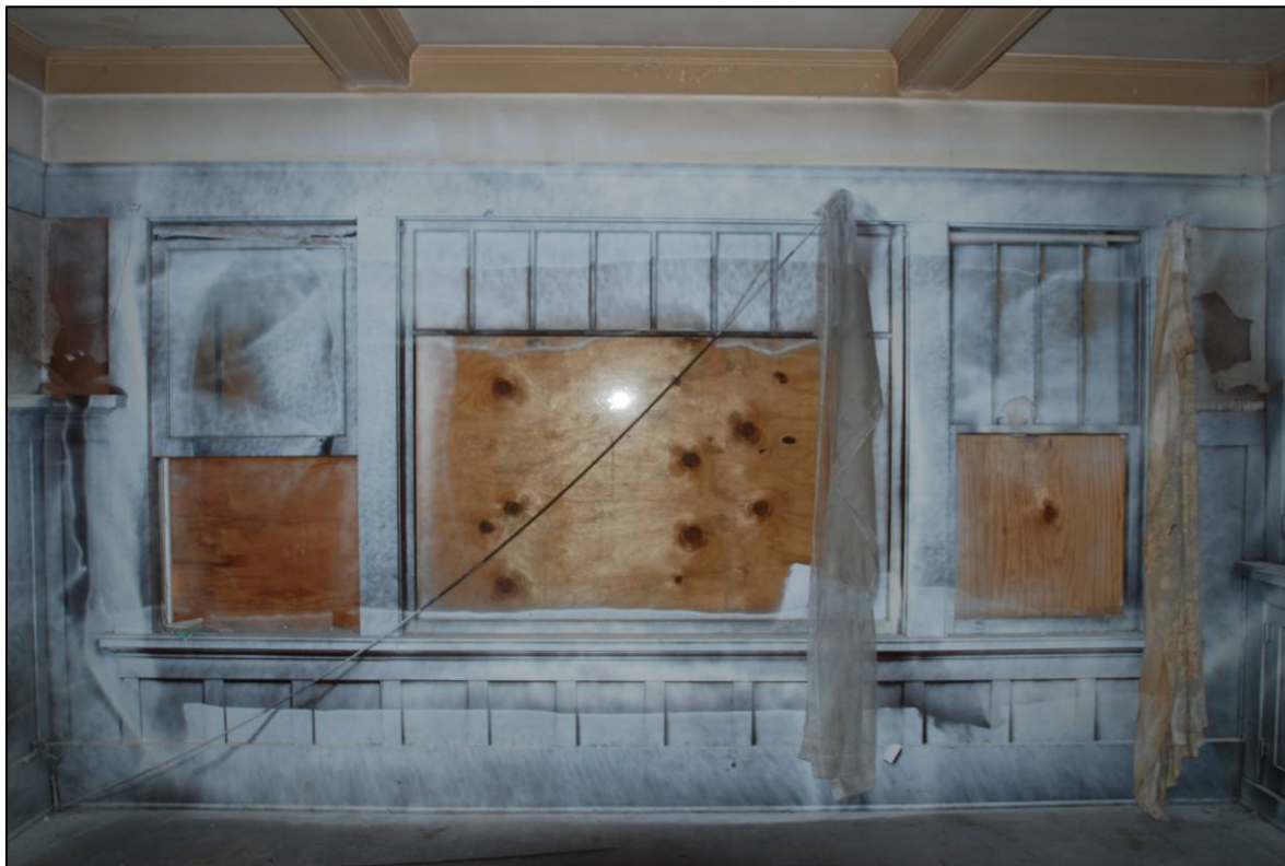
Photograph 22 South Side Window 3 Interior Shot
