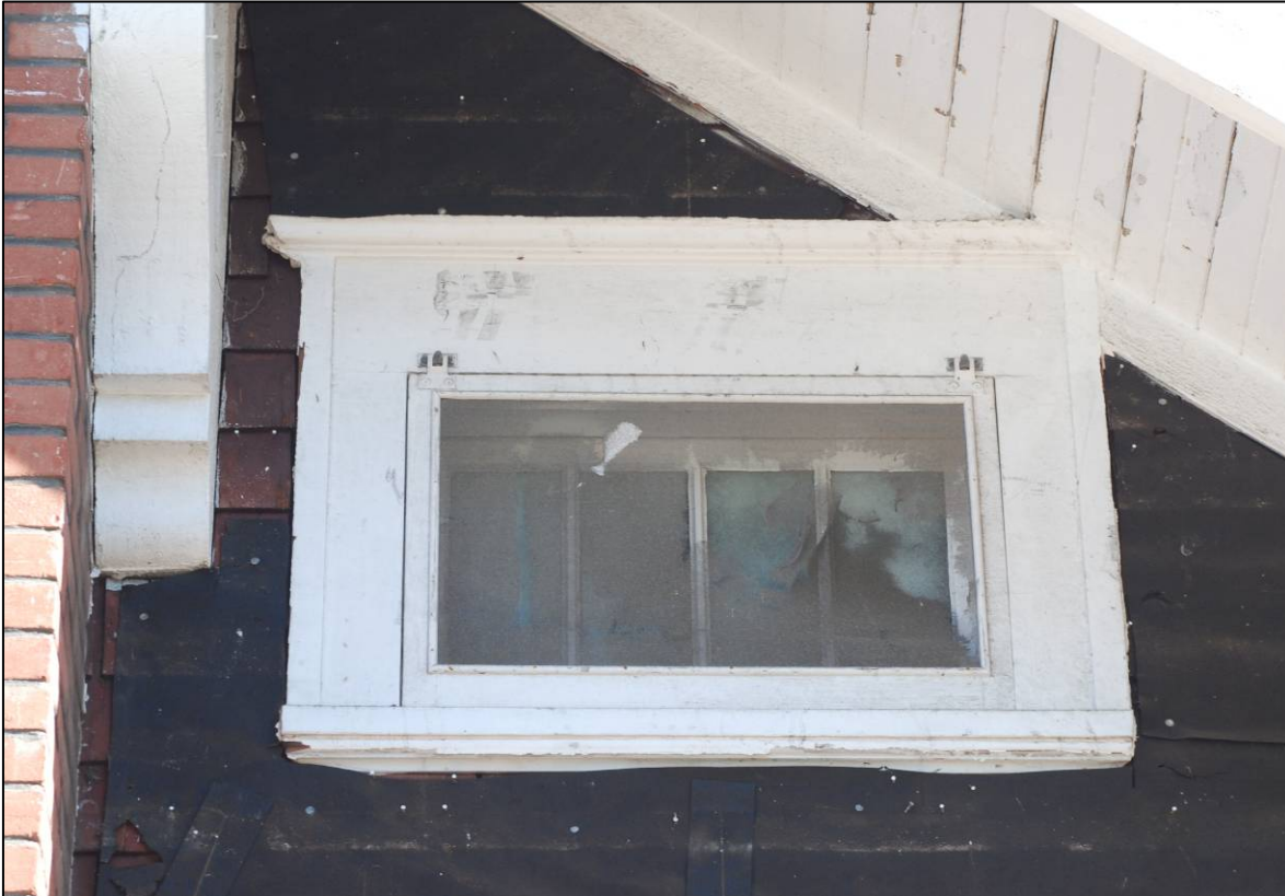
Photograph 23 Second Floor Top Hinged Window. Note typical main house window casing.
