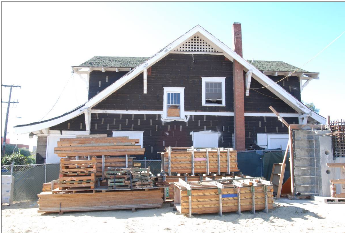
Photograph 4 North Side of House, Showing Location of Roof Curve Relative to Possible Front Porch
