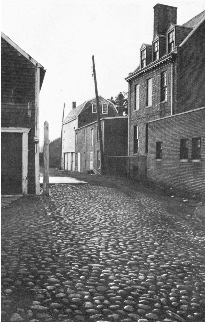
Without the cobblestone paving, the quality of the surroundings of the Steven's Wharf Buildings in Newport, R.I., would be greatly diminished. Photo by Jack E. Boucher, Sept. 1969. RI-304
