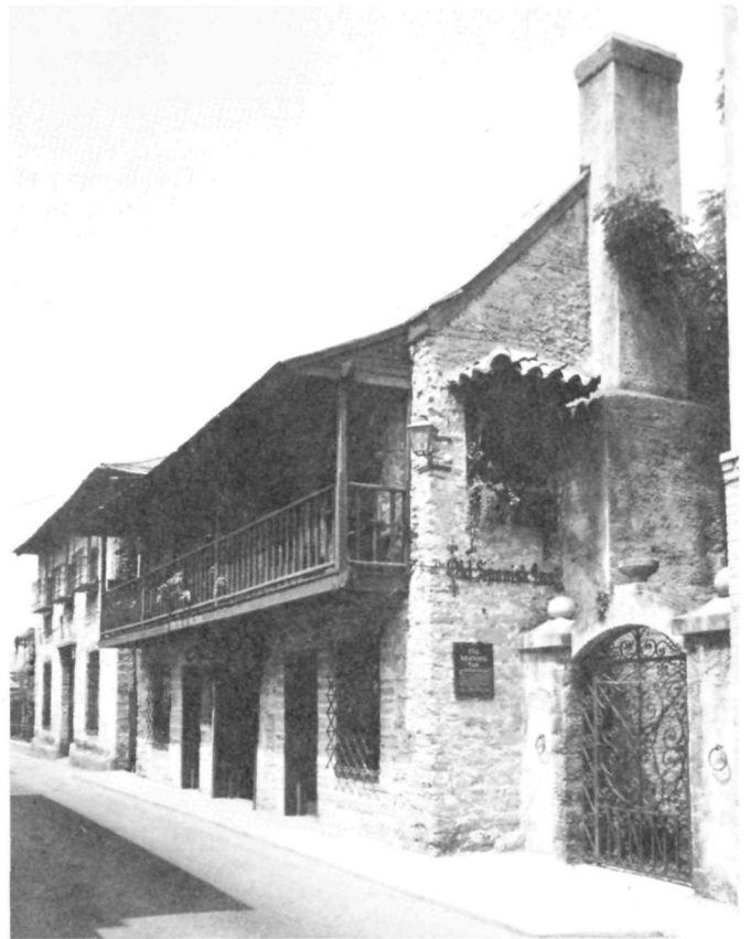
Built before 1764, the De Mesa-Sanchez House in St. Augustine, Fla., is an example of our Spanish architectural heritage. Although it has been altered and added to over the years, it still maintains its original character in the massive stone masonry construction, relieved by delicate wrought iron and overhanging balconies. Patio, from east (above). Photo by Jack E. Boucher, Feb. 1965. LC-NEG HABS FLA, 55-SAUG. 33-5
