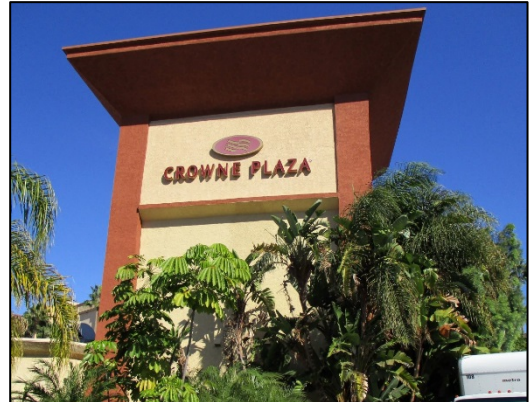
Figure 3: Antennas and equipment are all concealed within this tower element.
