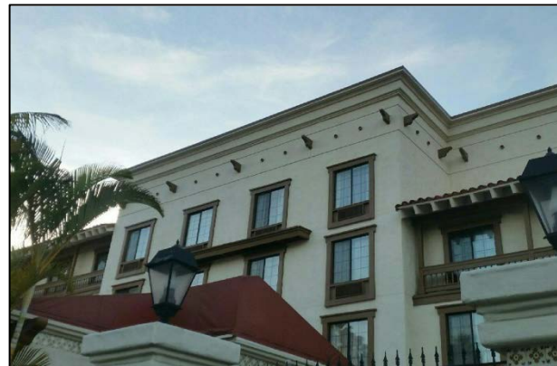
Figure 4: A completely concealed WCF. There are antennas in this picture!
