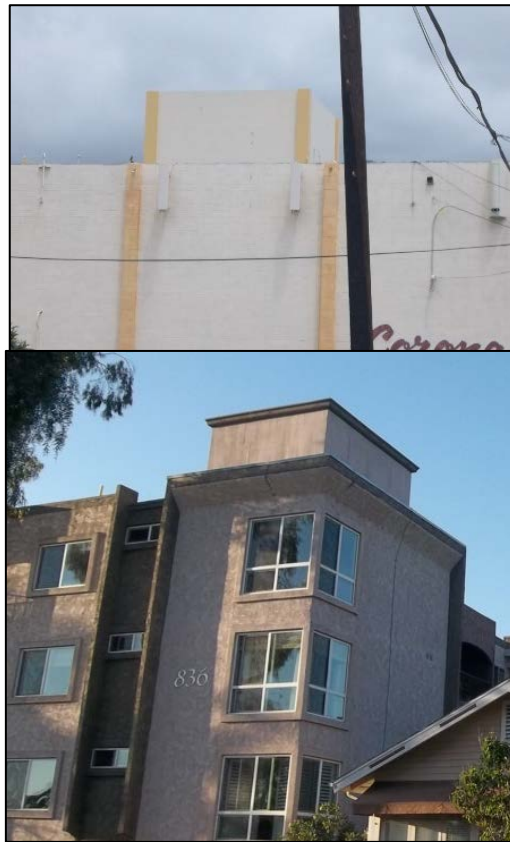
Figure 28: Two rooftop boxes that replicate existing building elements well.
