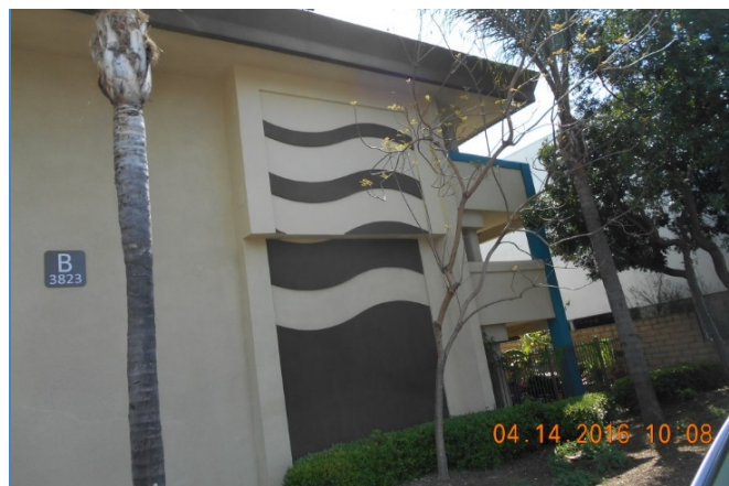
Figure 15: Although façade-mounted boxes are not preferred, this is still an excellent example of integration.
