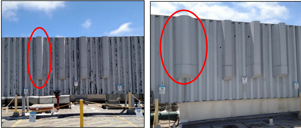
Figure 2: One sector of this site is balanced... ....and one sector is not.
