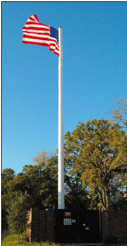
Figure 24: There are antennas in this flagpole.
