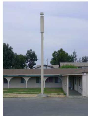
Figure 25: A parking lot light with an antenna shroud that complements the pole.
