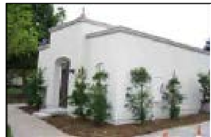
Figure 6: Equipment is concealed within this enclosure with the air conditioning units located on the roof behind the parapet.
