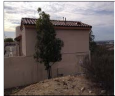
Figure 5: The generator is concealed inside the building above the existing equipment enclosure.
