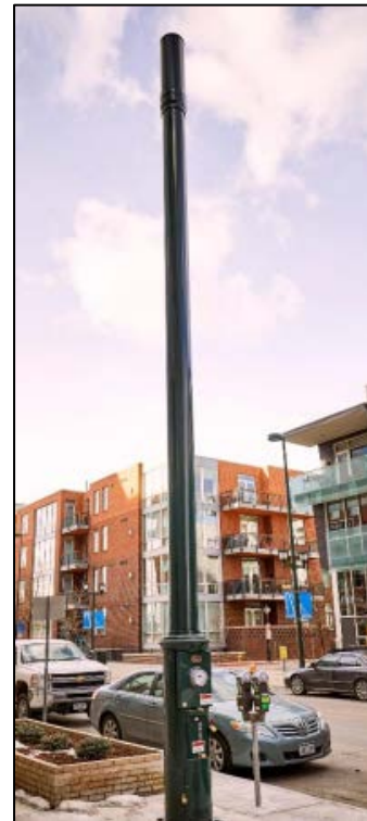
Figure 31: Stand-alone small cell pole in Denver, Colorado. Exposed utility meters are not preferred in San Diego.
