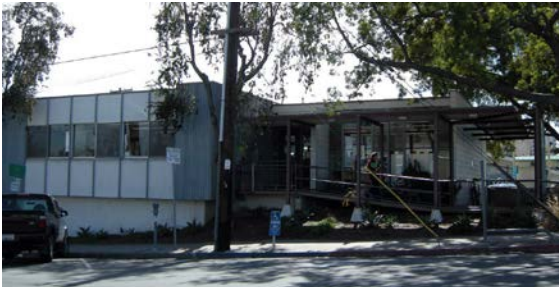
University Heights Branch Library, 4193 Park Boulevard.
