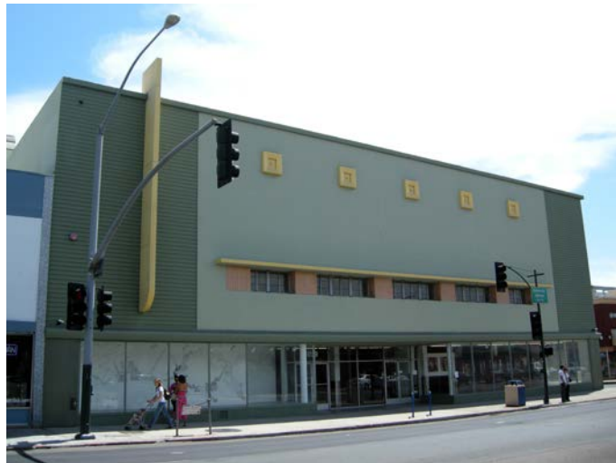
J.C. Penney Co. Building, 3029 University Avenue.
