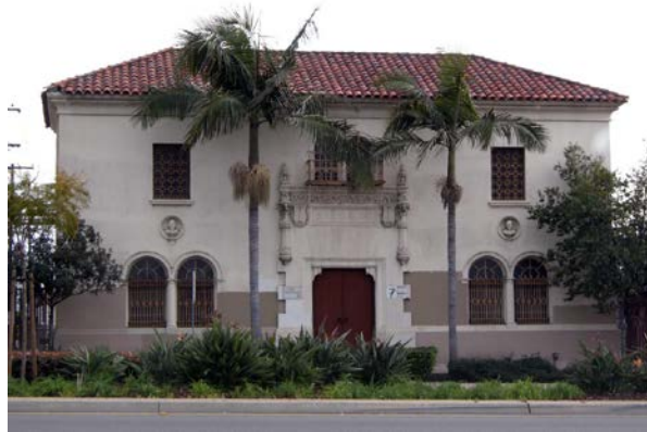
San Diego Gas & Electric Co. Substation F.
