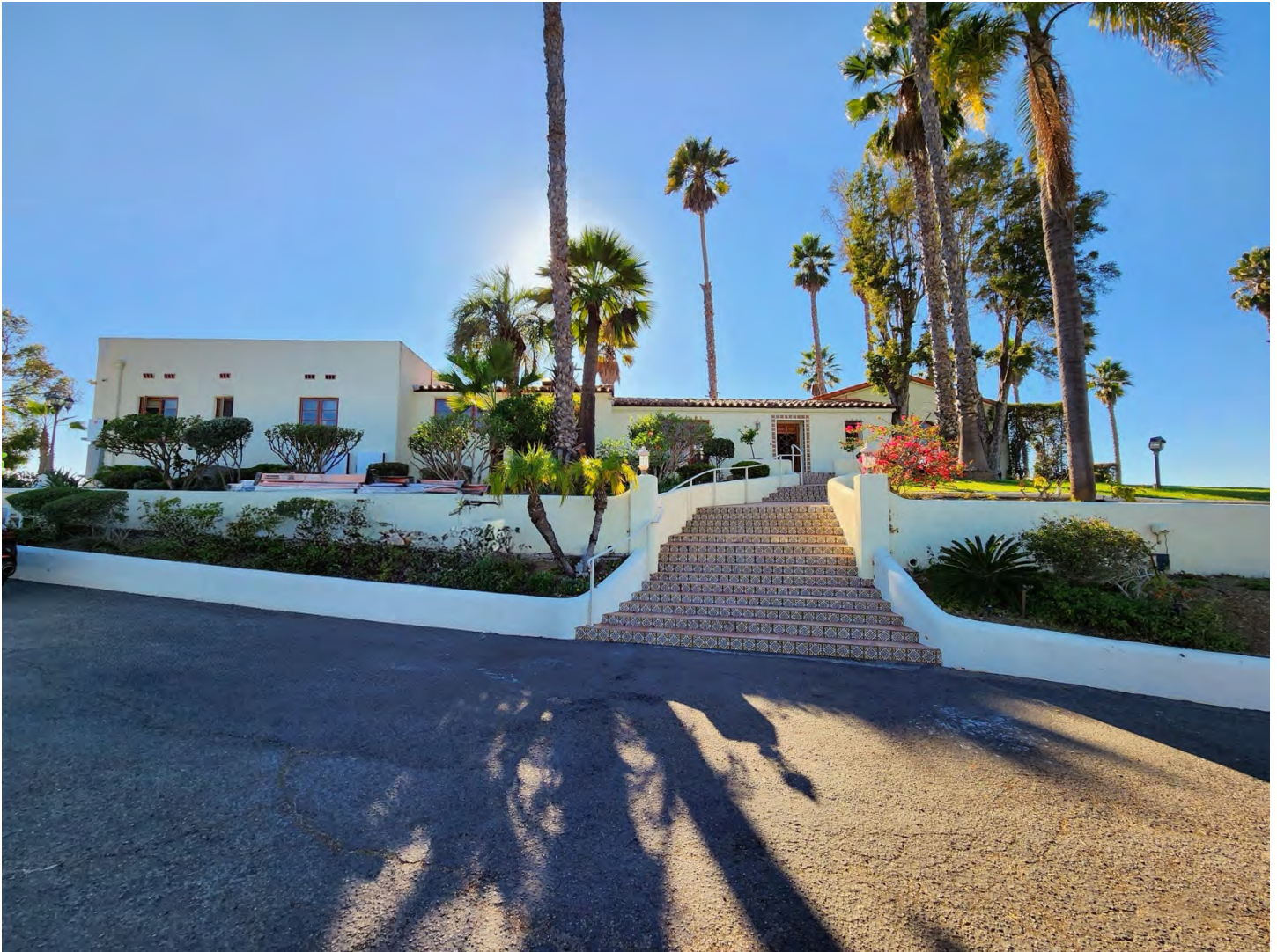
Photo 4: The residences is characterized by its elongated, irregular massing, smooth stucco walls, its low-pitched red clay tile roof, and a composition of intersecting volumes arranged around a private central courtyard. Source: Urbana Preservation & Planning, LLC.
