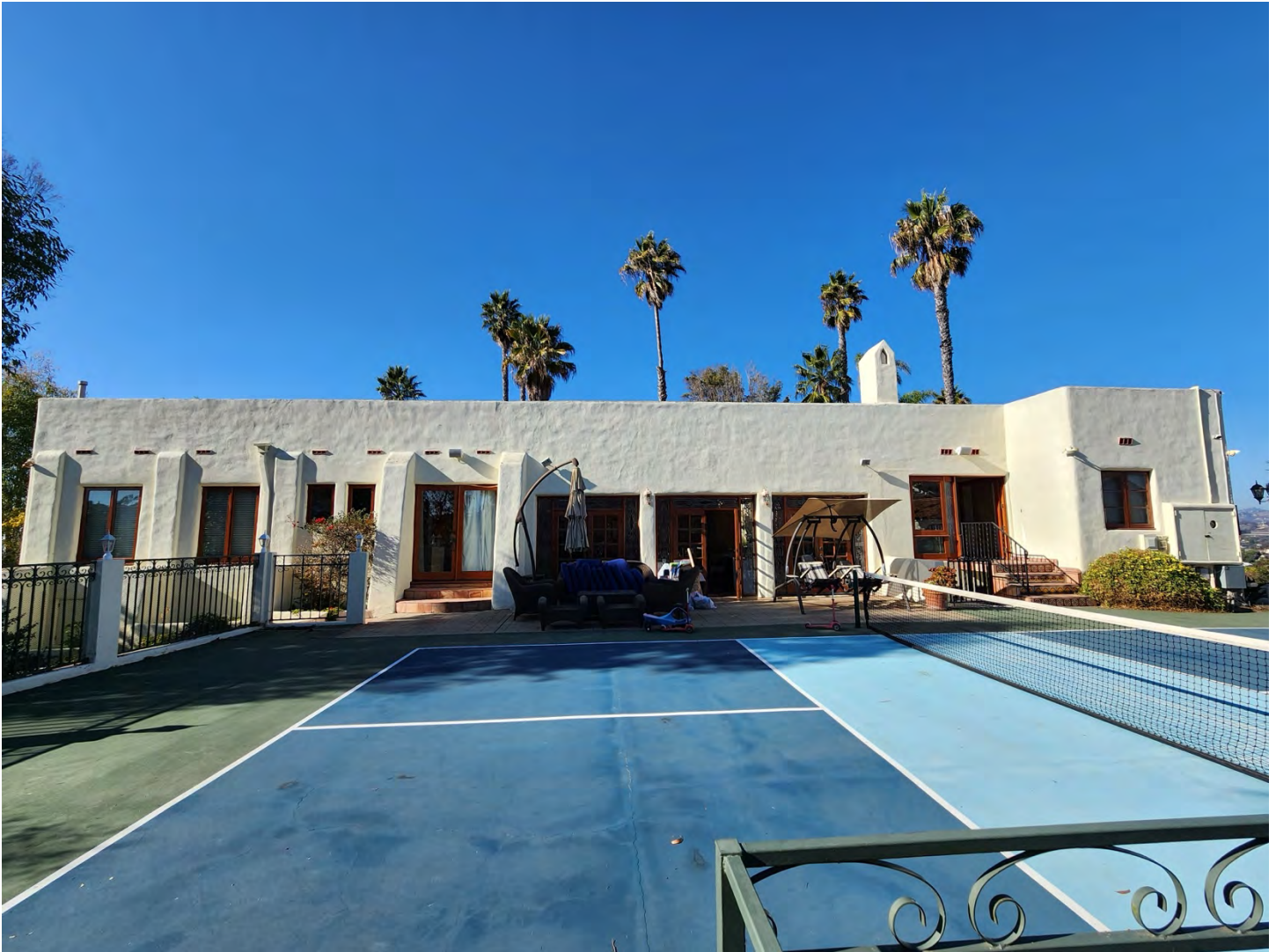
Photo 10: The south elevation includes the dwelling's flat-roofed section and features prominent stucco buttresses along the west side, a smooth stucco façade, low parapet roofline, and several rectangular single-lite casement windows of various sizes, all of which are replacements for the original multi-lite casements but remain within original openings.
