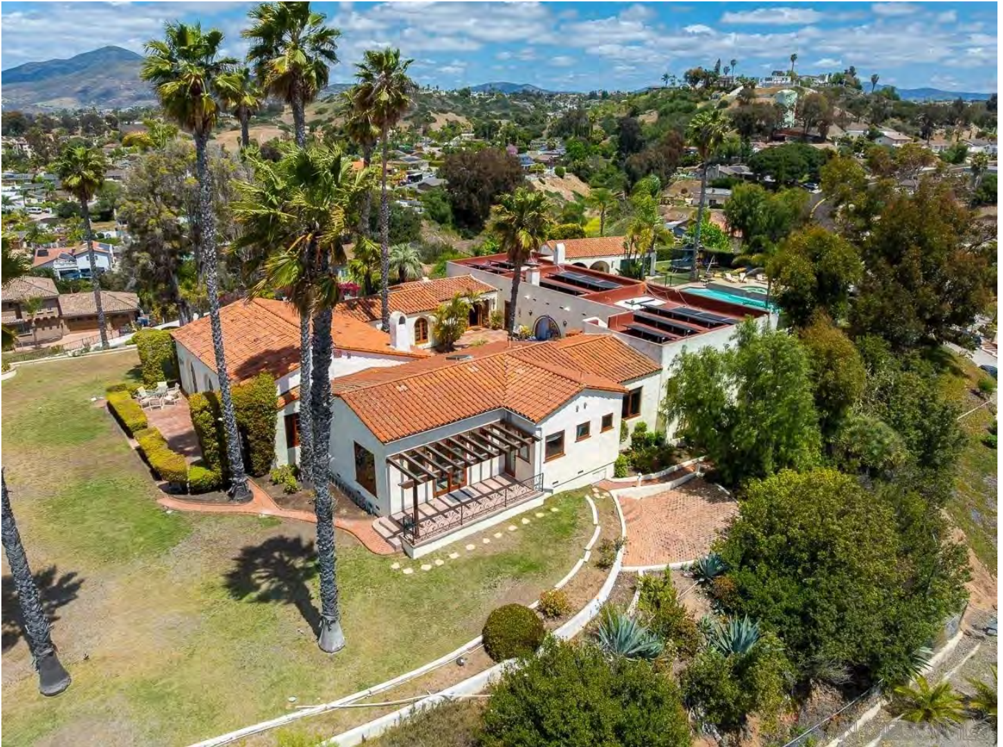
Photo 3: The residences is characterized by its elongated, irregular massing, smooth stucco walls, its low-pitched red clay tile roof, and a composition of intersecting volumes arranged around a private central courtyard. Source: Redfin.
