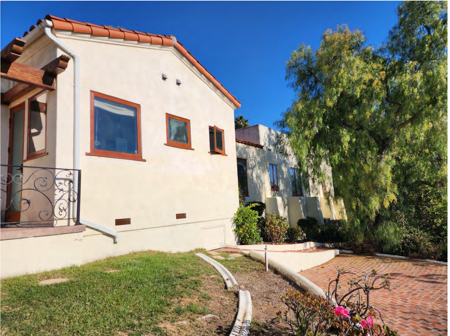
Photo 9a: South / right of the addition is the original west elevation which transitions to a small central portion with a clay tiled roof, followed by a flat-roofed section defined by regularly placed stucco buttresses. Source: Urbana Preservation & Planning, LLC.
