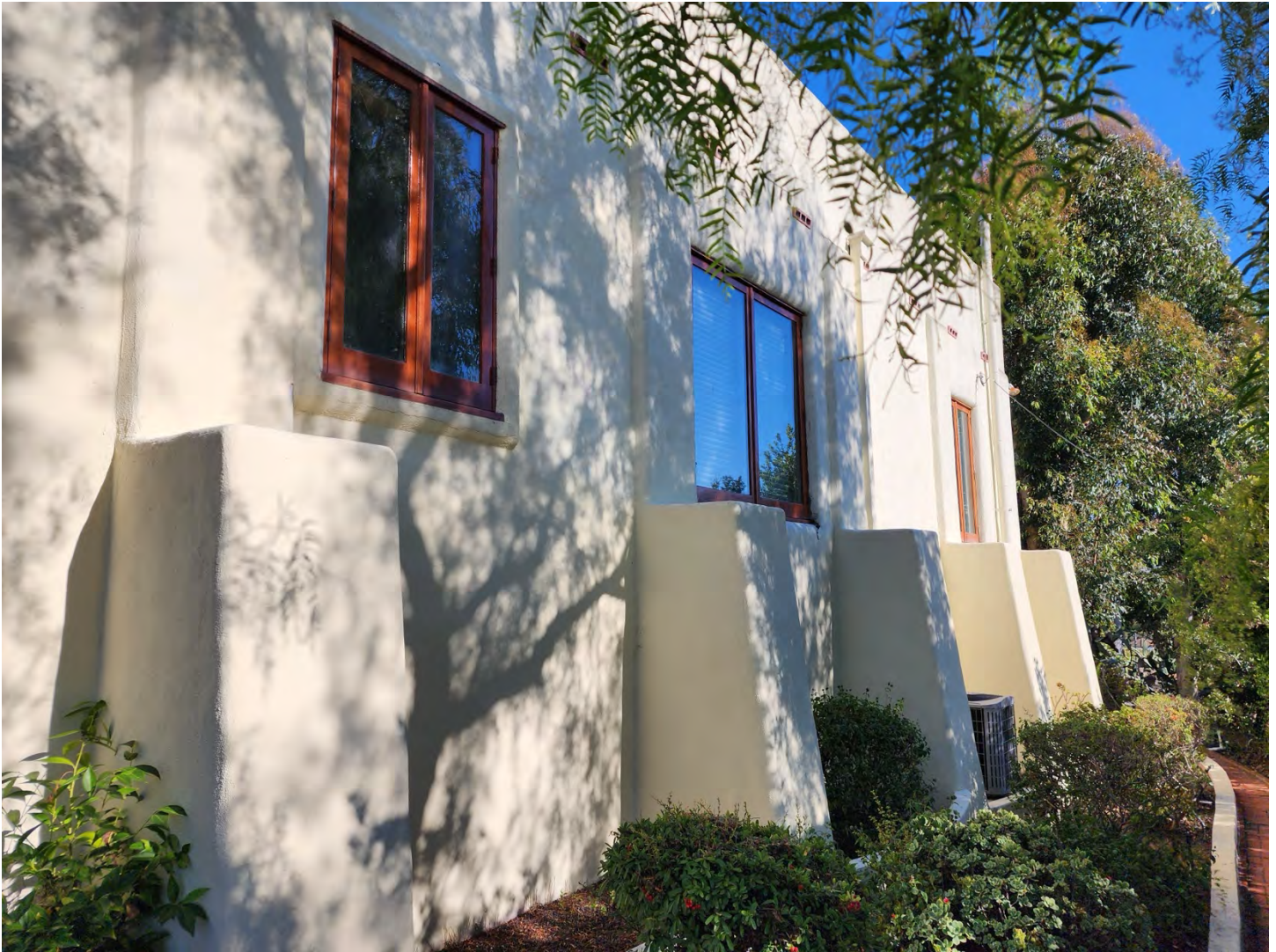
Photo 9c: West elevation buttresses. Source: Urbana Preservation & Planning, LLC.
