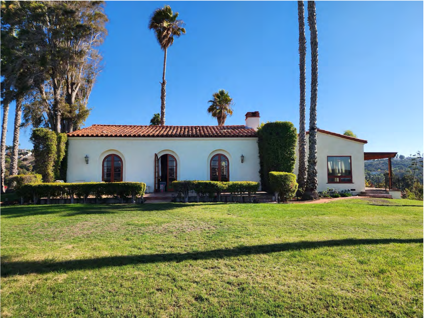
Photo 6: The north elevation faces La Cresta Way and neighboring property 3915 La Cresta Way. An addition, constructed in 2005, fills the west / right side corner.
