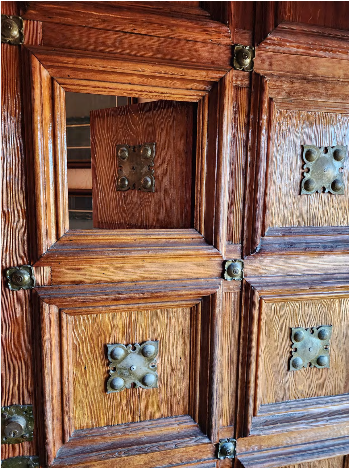
Photo 5b: The main entryway is set within a recessed opening, framed by decorative hand-painted tiles. The wood entry door, original to the dwelling, is highly detailed, featuring a geometric spindle work and ornamental metal accents. Source: Urbana Preservation & Planning, LLC.
