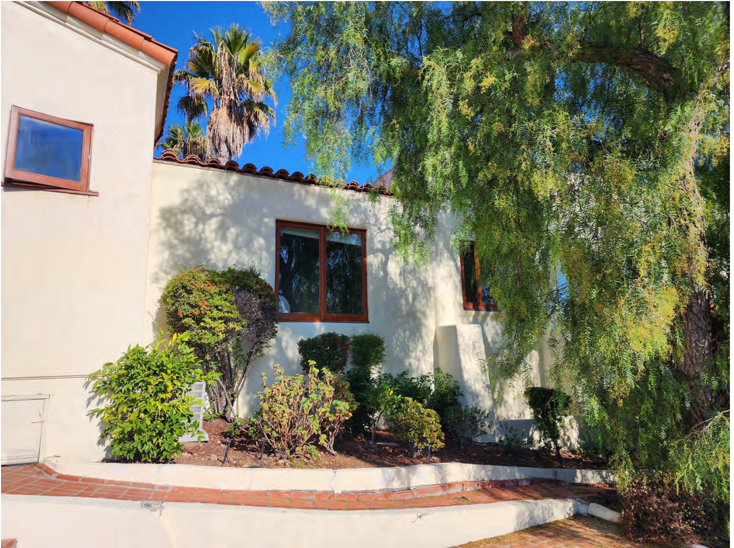
Photo 9b: West elevation. Source: Urbana Preservation & Planning, LLC.
