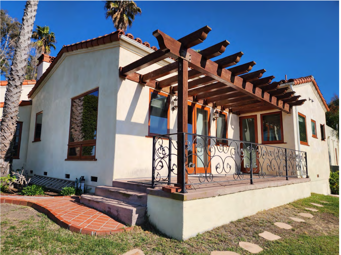
Photo 8: View of 2005 addition. The addition is characterized by a lower cross-gabled roof with red clay tiles, a pergola-topped patio and modern wood-framed glass doors and wood single-lite windows that complement the historic appearance of the property. Source: Urbana Preservation & Planning, LLC.
