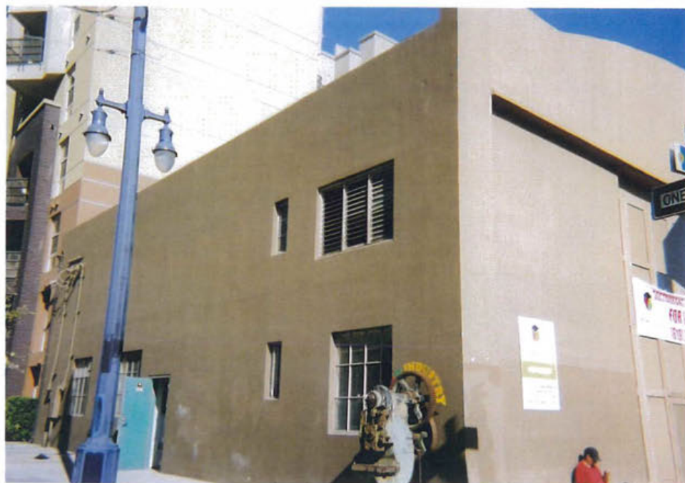
4. 1220 J Street View North/West Facade December 2007
