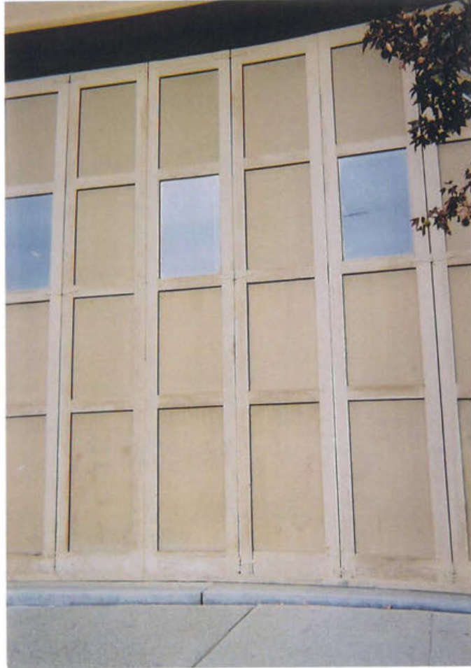
11. 1220 J Street/Door Detail View North/South Facade December 2007
