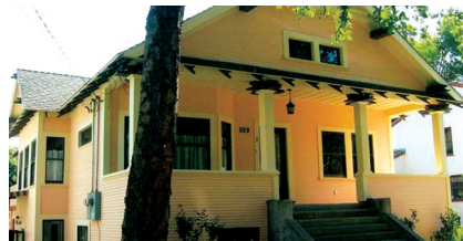
Above: A rehabilitated 1908 residential duplex, South of Campus Neighborhood National Register District, Chico. Top right: General Petroleum office building in Los Angeles, renamed The Pegasus, used tax credits in project financing.
