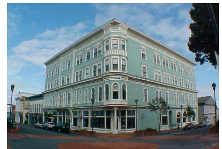
Built in the early 1870s, Eureka's Vance Hotel was wired for electricity by 1885. Restored and seismically stabilized, it houses retail, office, and commercial spaces.
