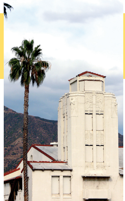
The Grand Central Air Terminal, 1310 Air Way in Glendale is a currently active 20% Federal tax credit project.
