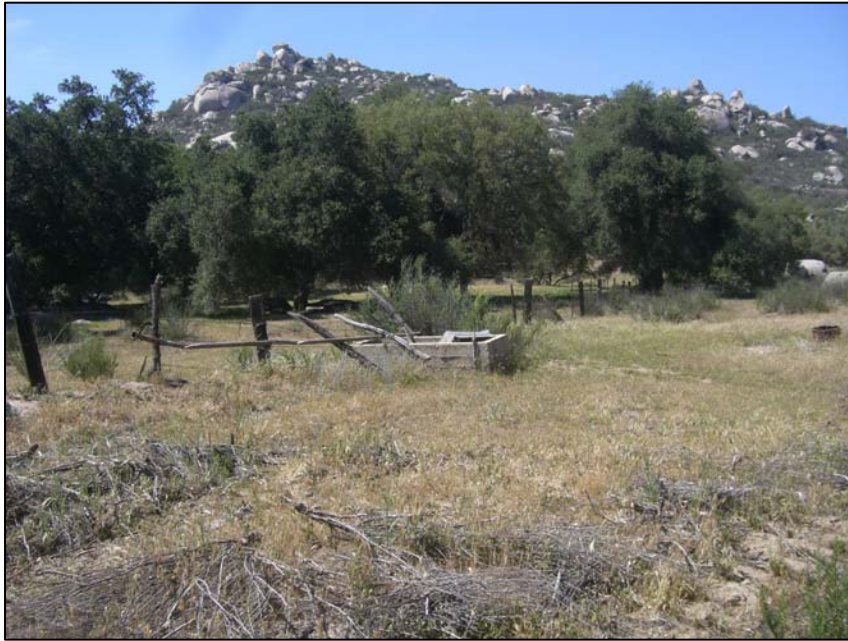
Concrete trough at Round Potrero.
