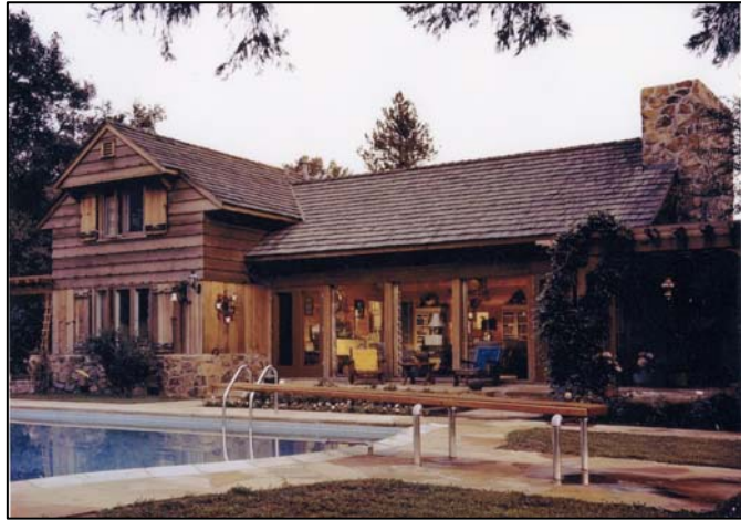
Ranch house designed by Charles Luckman
