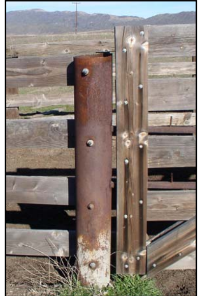
Upright made from used well casing.
