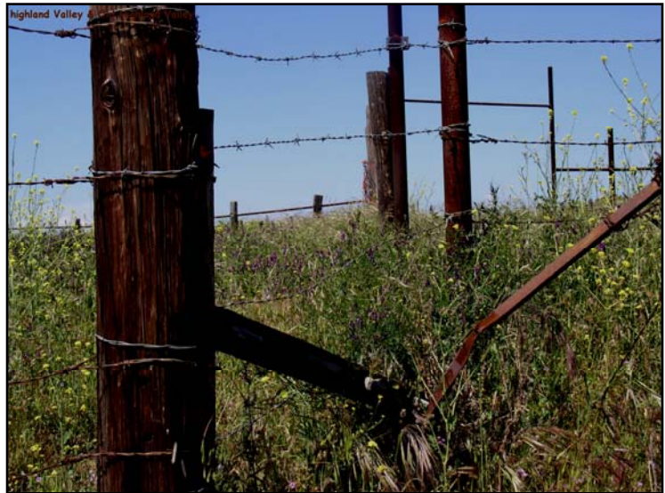
Power pole with insulator posts still attached.
