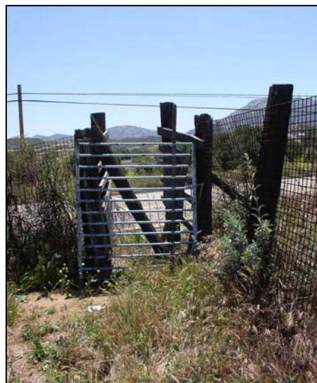
Blocking gate to restrict cattle access.
