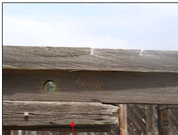
Power pole used as horizontal beam.
