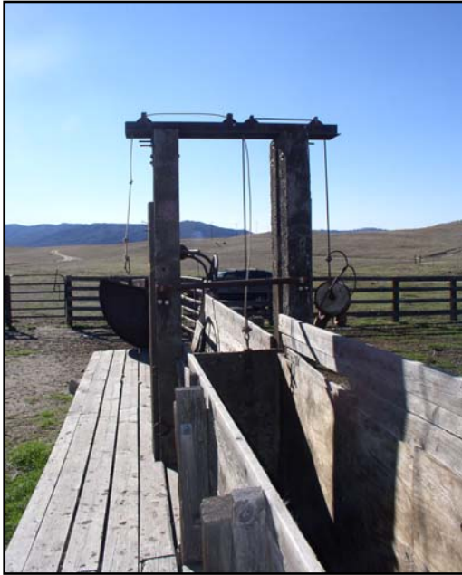
Working chute and head gate (guillotine) with catwalk in left side of photo.
