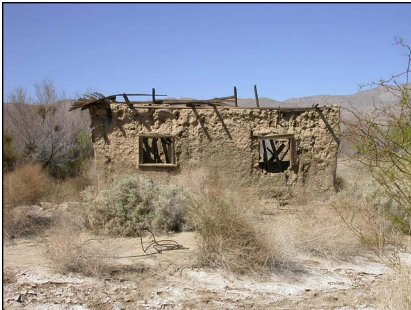
Bailey earthen structure - 2003
