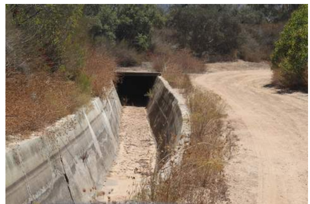
The conduit follows along Flume Road before meeting Dulzura Creek
