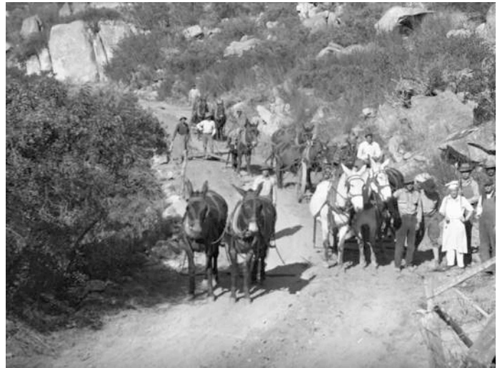
Supplies for the construction of Barrett Dam came by way of Lyons Valley Road, 1920
