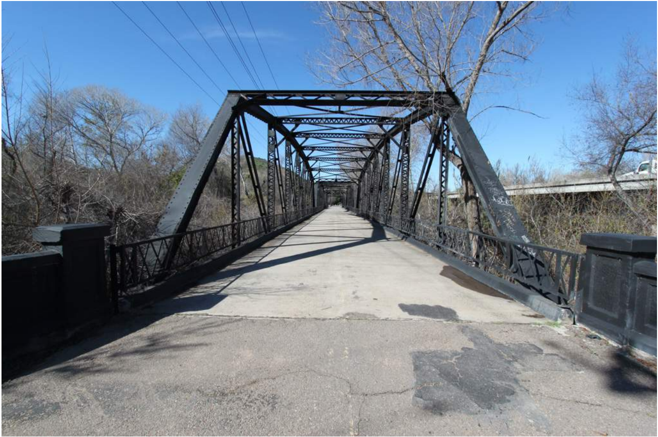
Sweetwater River Bridge
