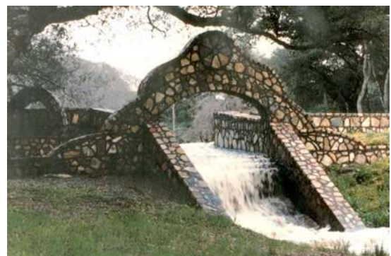
Dam and spillway east of the Post.
