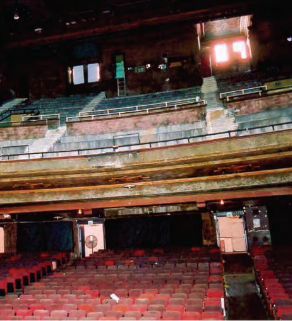
Above The interior of the theater in 2000, prior to restoration. Note the patchwork of non-historic seats and the heavily tarnished walls. The CCDC deserves much credit for keeping the building watertight and free from vagrants during its 20-year hibernation.
