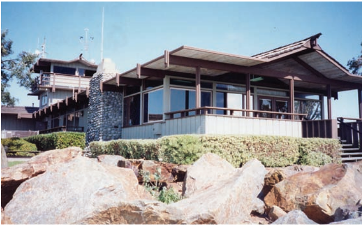
Mission Bay Aquatic Control Center, designed by Sim Bruce Richards, 1960. Photo by Keith York, 2004.
