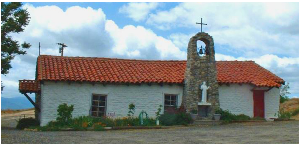
View showing the south wall of the 1830s Saint Francis Chapel in Warner Springs that SOHO volunteers restored in 1994 after it had sustained damage during one of the longest periods of consecutive days of rain on record. One of many historic sites in San Diego County. Photo by Lisbeth A. Christensen, 2005.
