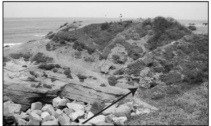
Cobblestone anchor for historic bridge.
