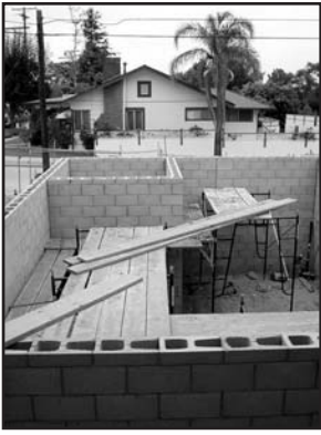
An 8' high block foundation, the beginning of a MacMansion
