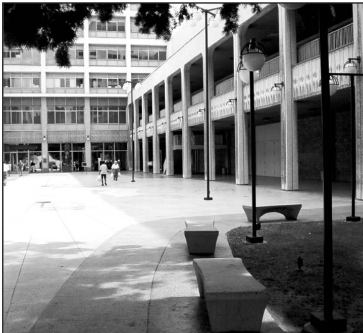
San Diego Community Concourse, 1964. Designed by Tucker, Sadler and Bennett.
