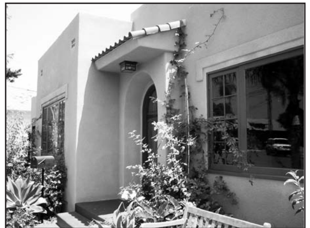
Example of correct stucco on this 1926 Craftsman Bungalow.
