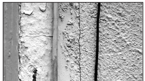
Example of poor restucco job. Stucco on this 1922 Spanish Revival is completely flush with window trim on left, different textures have been applied throughout the years.
