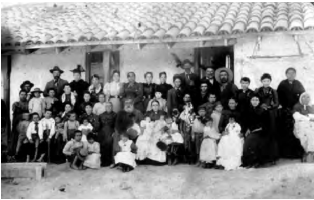
MARRON ADOBE - One of San Diego's earliest survivors of the Rancho period, located in Oceanside. The proposed new freeway entrance for Route 78 will encroach and threaten the integrity of this adobe, changing its historic landscape after 150 years. Ecological and archeological sites on or near the property will also be destroyed.
