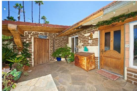
The adobe builders were building environmentally friendly 'green' homes well before the current trend, as most of the homes were built with the bricks made on site with a formula required at the time, using some asphalt stabilizers for waterproofing and some cement for strength. The thermal properties of adobe (16-inch-thick walls) mean less energy use for heating and cooling.
