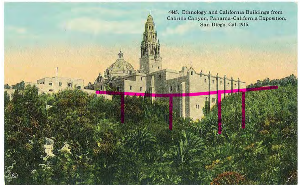
Figure 11 - Same view as Image 14 showing the proposed Bypass Bridge and column supports in pink from Cabrillo Bridge to Alcazar Gardens.
