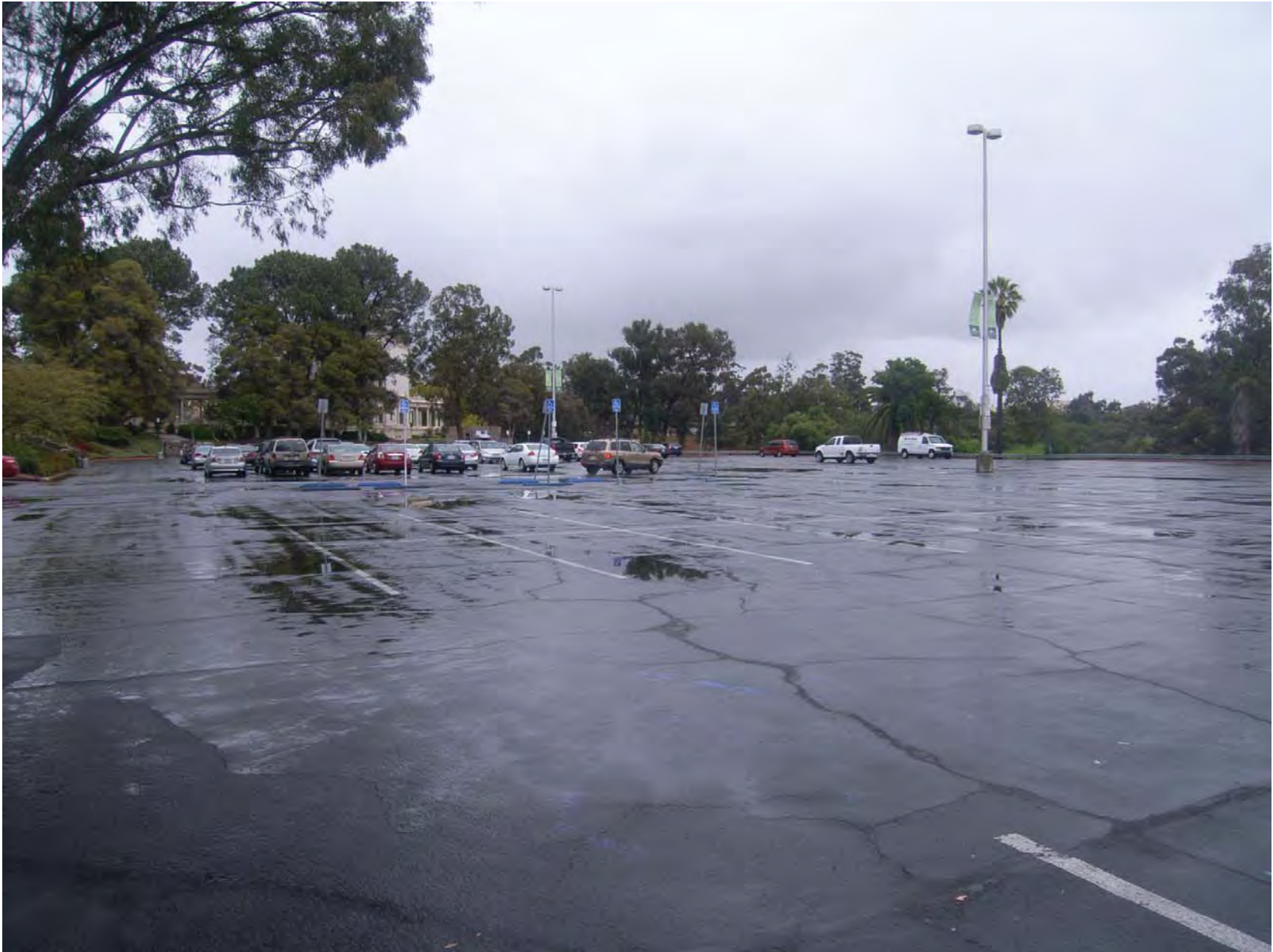
FIGURE 4.3-7 Organ Pavilion Parking Lot
