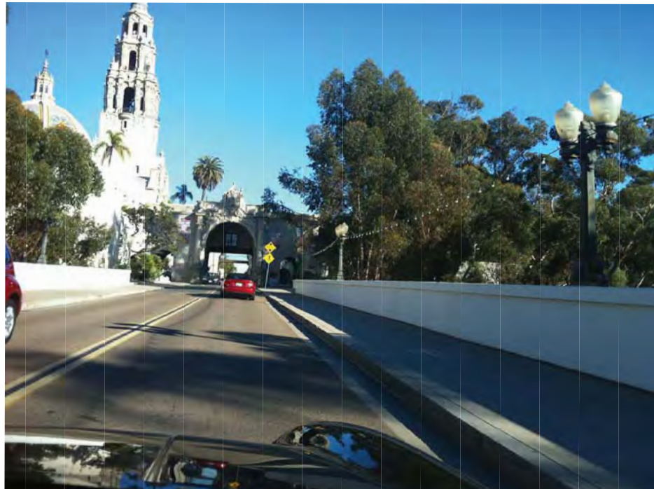
LIGHT SAND FINISH/STUCCO RETAINING WALL
