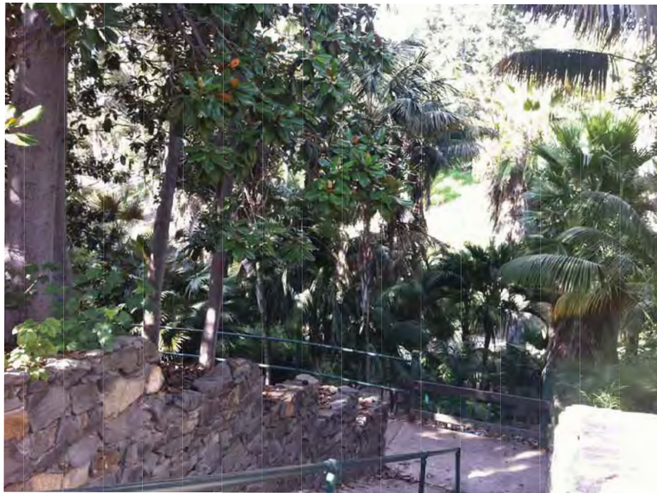
STACKED STONE RETAINING WALL
