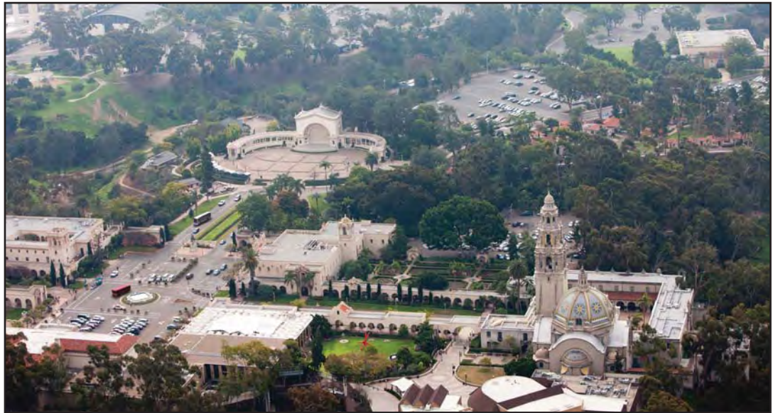
Existing Parking Lot from North
