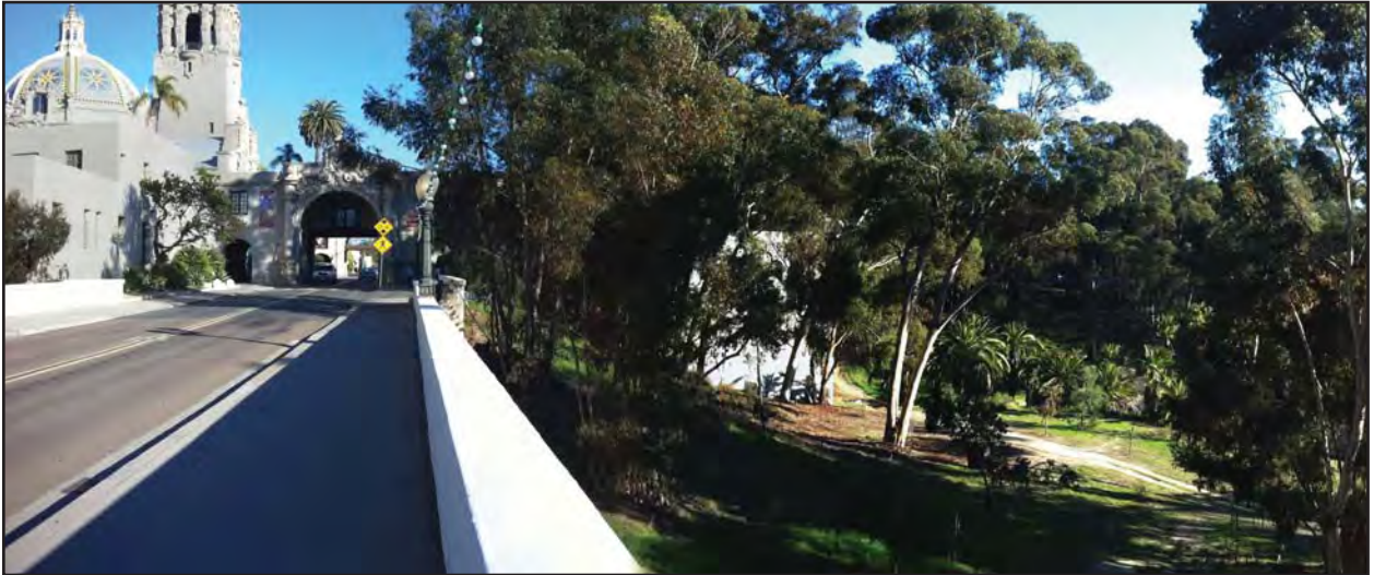
View of Cabrillo Bridge without Centennial Bridge
