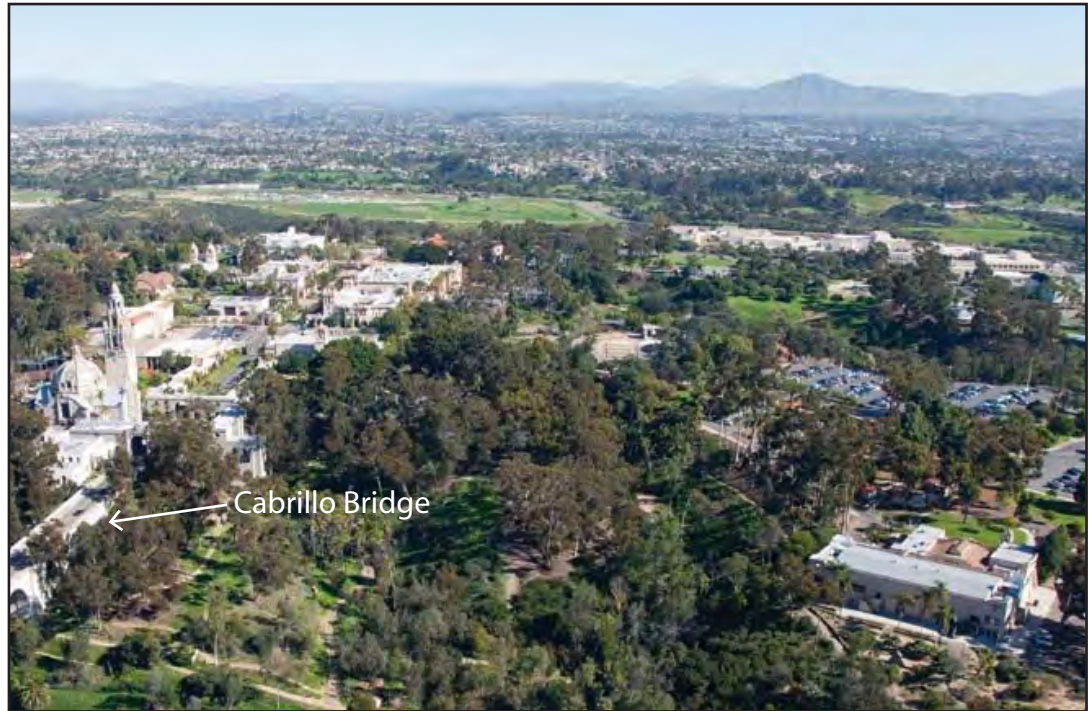
View of Cabrillo Bridge without Centennial Bridge
