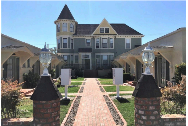
4270-4273 Campus Avenue. Courtesy San Diego Bungalow Courts and Apartment Courts Historic Context Statement
