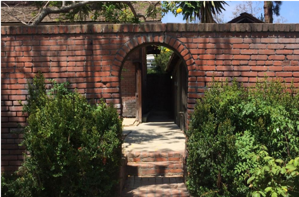
Above Photo - High brick garden walls on the west and north sides of the 1928 formal garden. The west wall separated the 1928 Formal Garden from functional property uses. The north wall separated the properties between the Marston's property and that of the Burnhams and Marston's son Arthur's homes.
