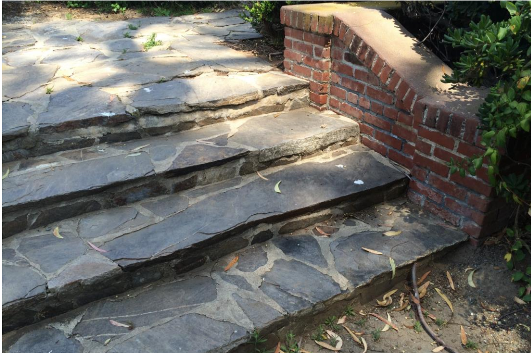
Above Photo - Indigenous Ramona granite staircase with brick cheek walls, from the 1928 Formal Garden period. Originally lawn separated the granite steppers, they now have cement mortar.
