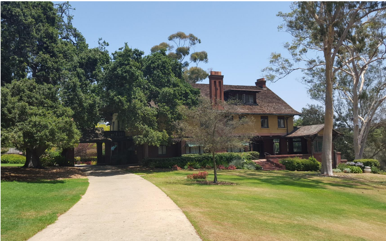
Photo 3 - Concrete Driveway toward Porte Cochere
